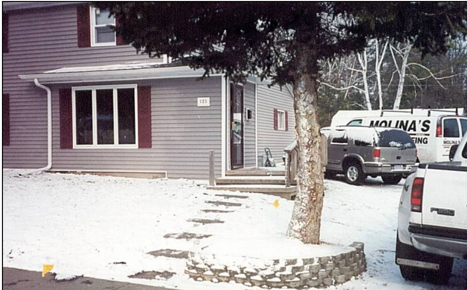
Figure 8-1. Residence before elevation
