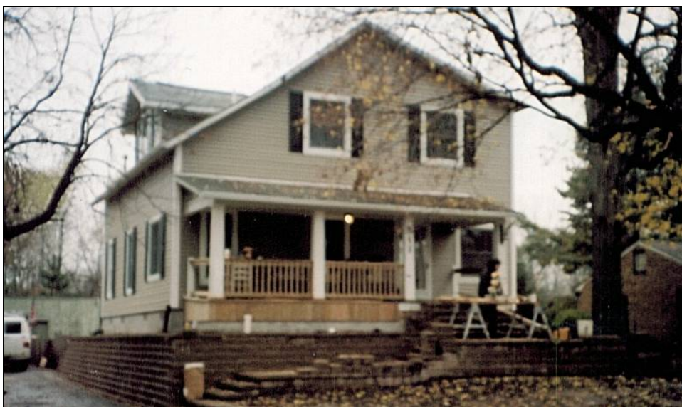
Figure 8-9. House elevated over 5 feet with retaining wall, porch, and landscaping
