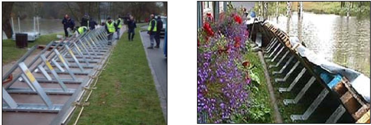
Figure 5-5. Metal supports for floodwall installed for deployment. Floodwall deployed with impermeable membrane.
