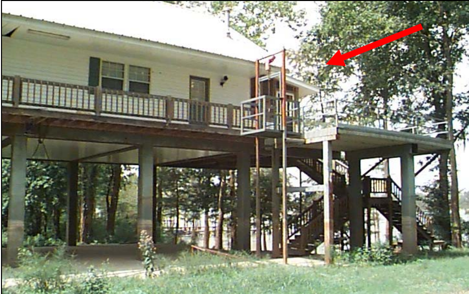
Figure 8-6. Elevator provides access to elevated structure
