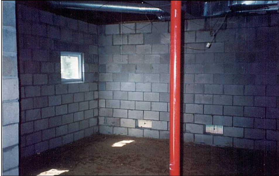
Figure 8-4. New foundation with vents
