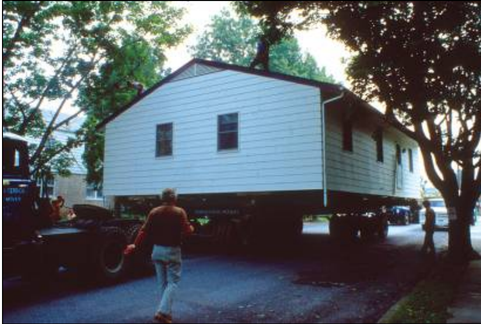
Figure 9-1. Structure placed on a wheeled vehicle for relocation to a new site
