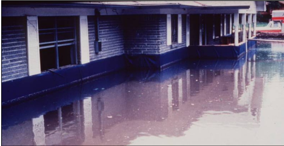
Figure 7-2. Photograph of membrane providing flood protection
