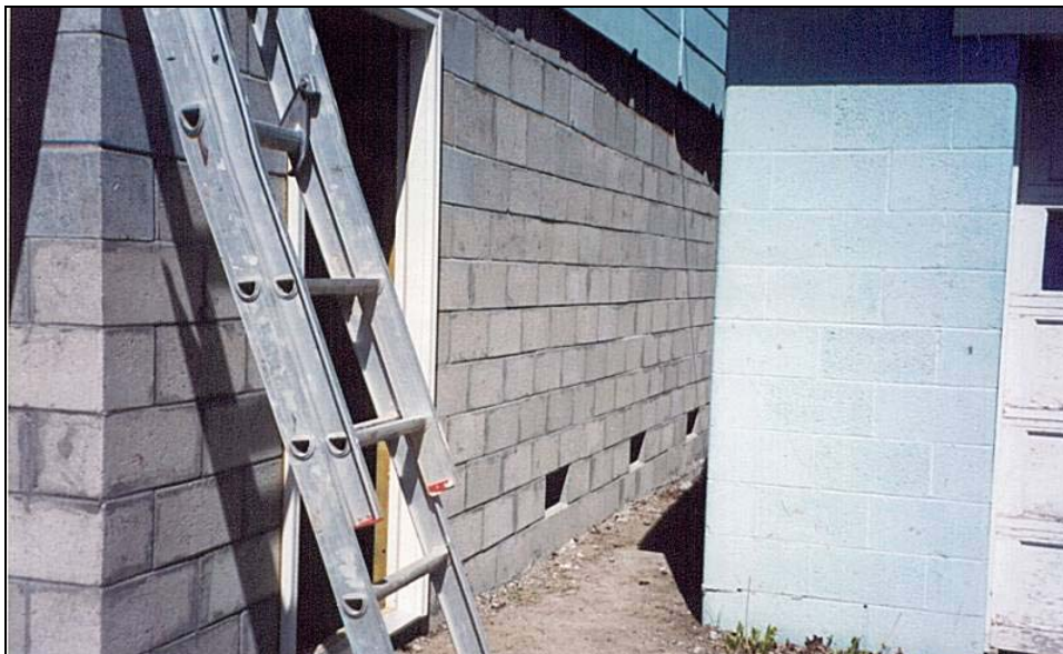
Figure 8-3. New foundation with vents
