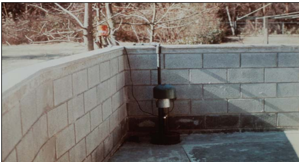
Figure 5-7. Small patio floodwall with sump pump
