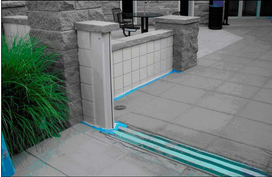
Figure 5-6. The City of Boulder, Colorado, installed a “pop up” closure to this floodwall at a City office building subject to flash floods. The closure floats up into place automatically when the site is flooded.
