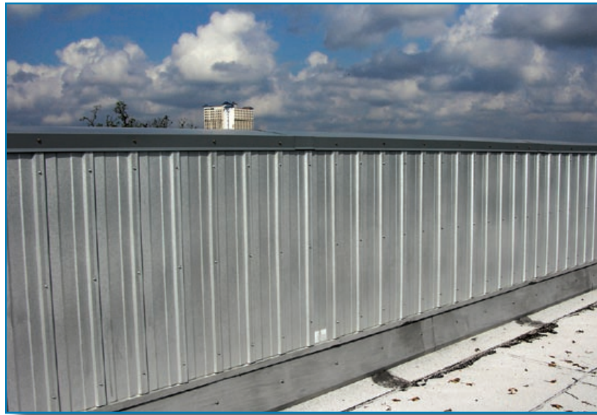
Figure 3-93: Base flashing protected by metal panels attached with exposed screws. Hurricane Katrina (Mississippi, 2005)
