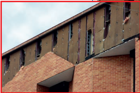
Figure 3-46: This tie remained embedded in the mortar joint while the smooth-shank nail pulled from the stud.
