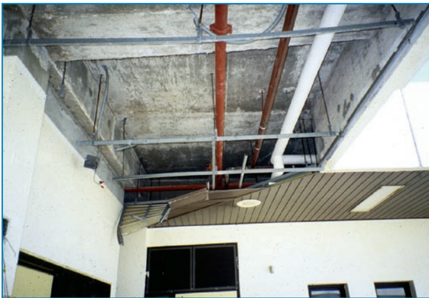
Figure 3-42: This suspended metal soffit was not designed for upward-acting wind pressure. Typhoon Paka (Guam, 1997)
