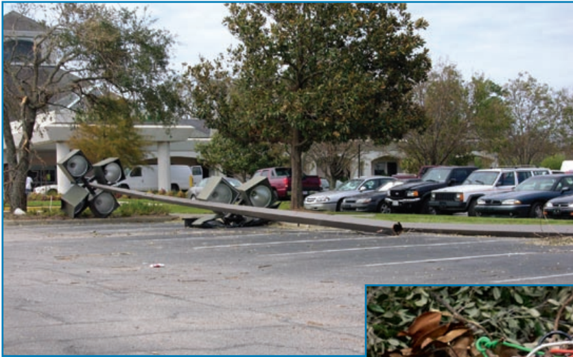
Figure 3-78: Collapsed hospital light fixtures caused by severe corrosion (see inset). Hurricane Ivan (Florida, 2004)
