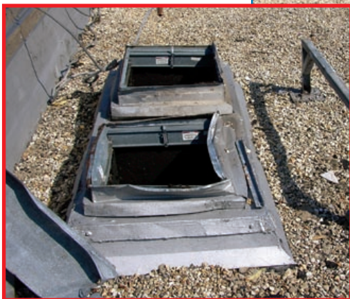
Figure 3-72: Two large openings remained (circled area and inset to the left) after the ductwork on this roof blew away. Hurricane Katrina (Mississippi, 2005)
