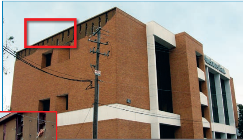
Figure 3-45: The brick veneer failure on this building was attributed to tie corrosion. Hurricane Ivan (Florida, 2004)
