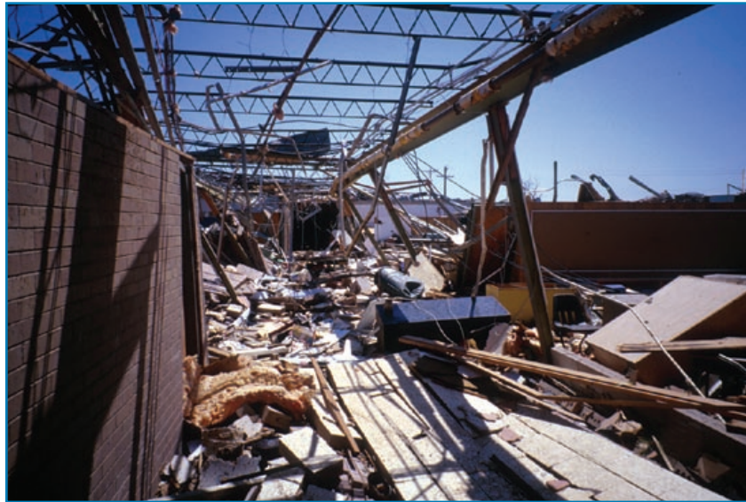
Figure 3-104: View of school corridor after passage of a violent tornado (Oklahoma, 1999)
