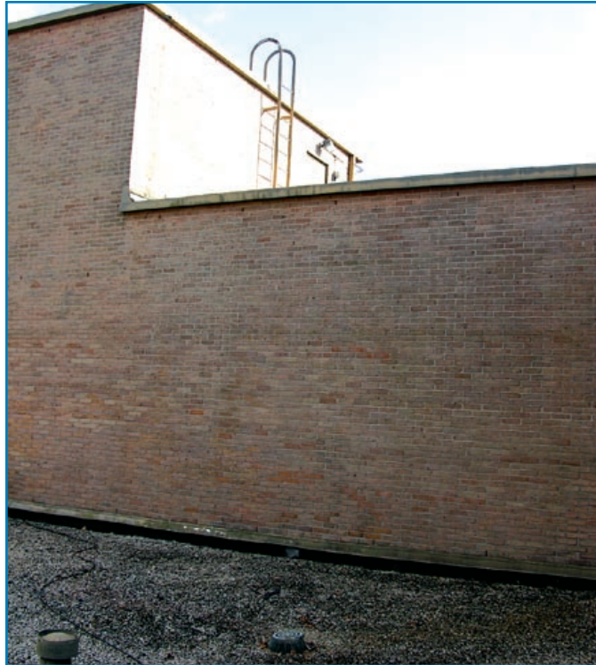
Figure 3-52: Water leaked inside along the base of the brick veneer walls. Hurricane Katrina (Louisiana, 2005)
