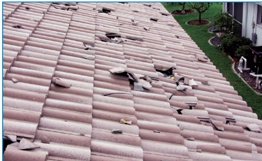
Figure 3-88: Brittle roof coverings, like slate and tile, can be broken by missiles, and tile debris can break other tiles. Hurricane Charley (Florida, 2004)
