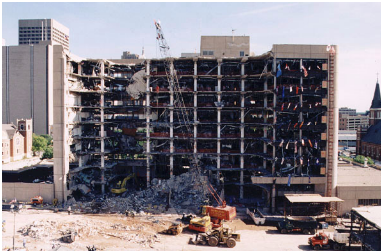
Figure 4-3 Exterior view of Alfred P. Murrah Federal Building collapse
