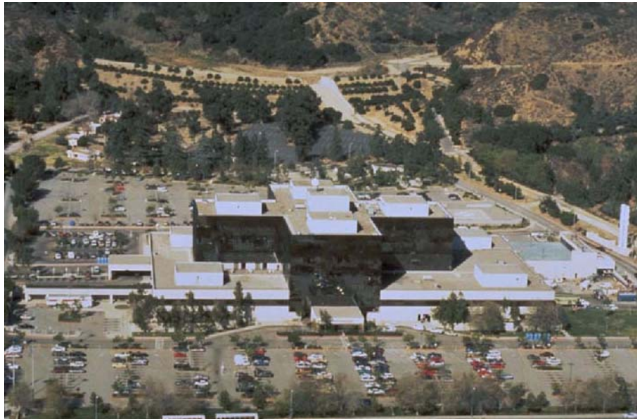
Figure 9-2 Aerial view of Olive View Hospital, which sustained no structural damage during the 1994 Northridge earthquake, but was closed for a short while after the earthquake because of water leakage from broken sprinklers and waterlines. (photo courtesy of the Earthquake Engineering Research Institute)
