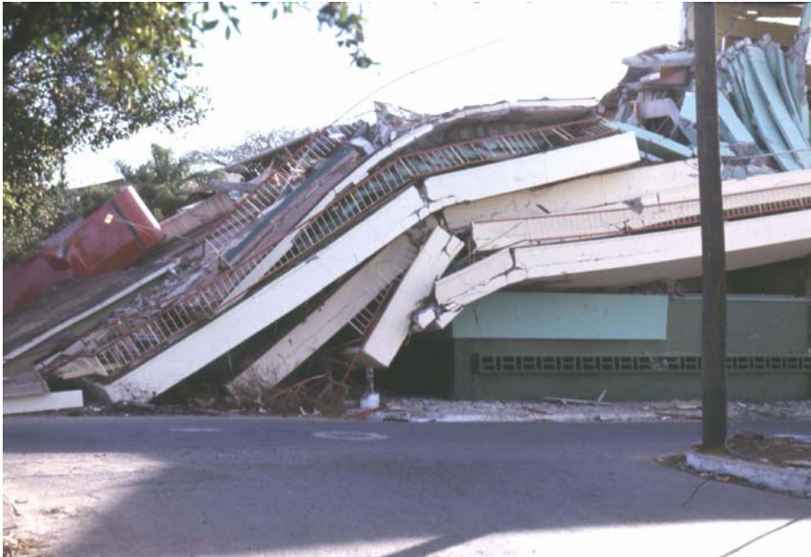
Figure 3-3 Older five-story reinforced concrete frame building in Managua, Nicaragua, that had inadequate seismic resistance and collapsed during the magnitude-6.2 earthquake of December 23, 1972. (photo courtesy of C. Rojahn)
