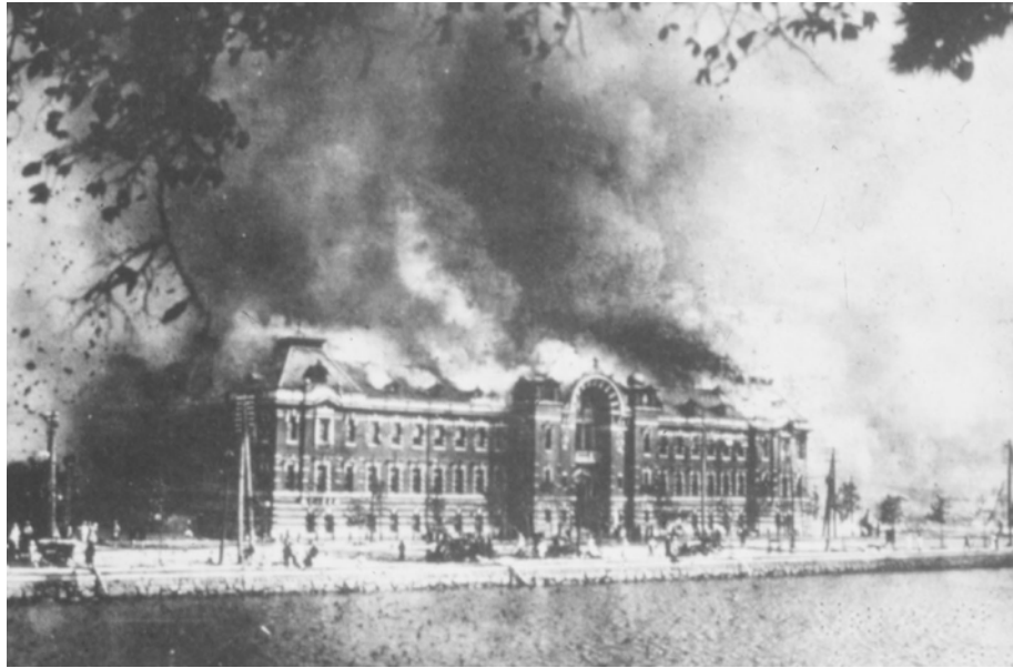
Figure 3-14 Photo showing the burning of the Tokyo Police Station following the magnitude-8.3 Tokyo/Kanto earthquake of 1923.
