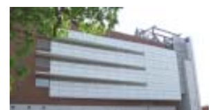
Building 11 - Power Plant
