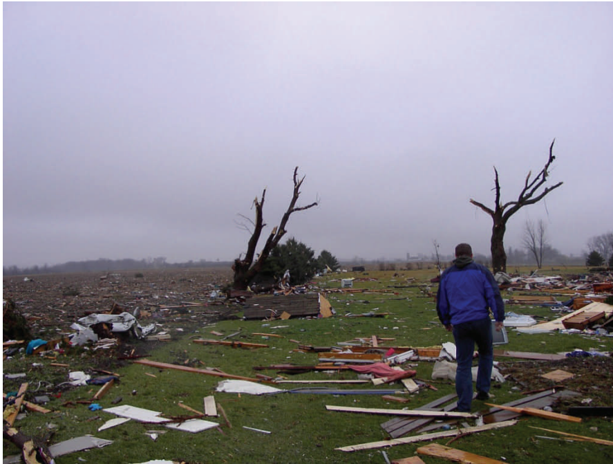
NWS meteorologist evaluates tornado damage in Boone County, January 2008 – NWS photo
