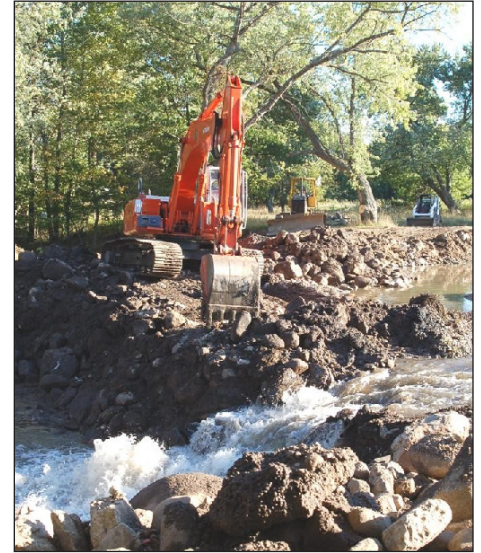
Hersey dam removal, MI
