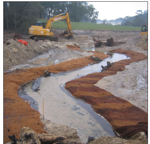
Restoration of 2,500 feet of stream channel in Mill Creek, FL for a self-sustaining population of endangered Okaloosa darters.
