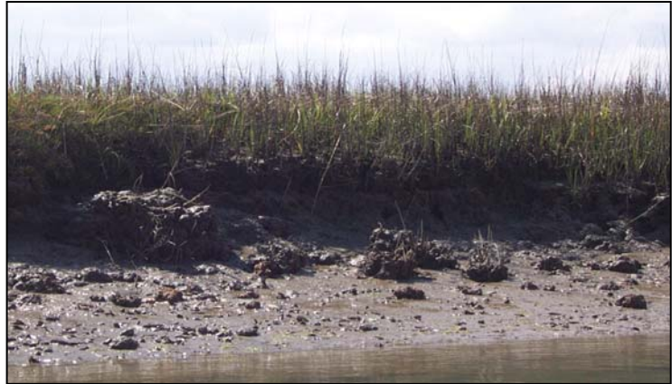
Figure 16. As marsh banks erode, blocks of mud and cordgrass drop onto the fringing bank where their appearance is similar to oyster reef.
