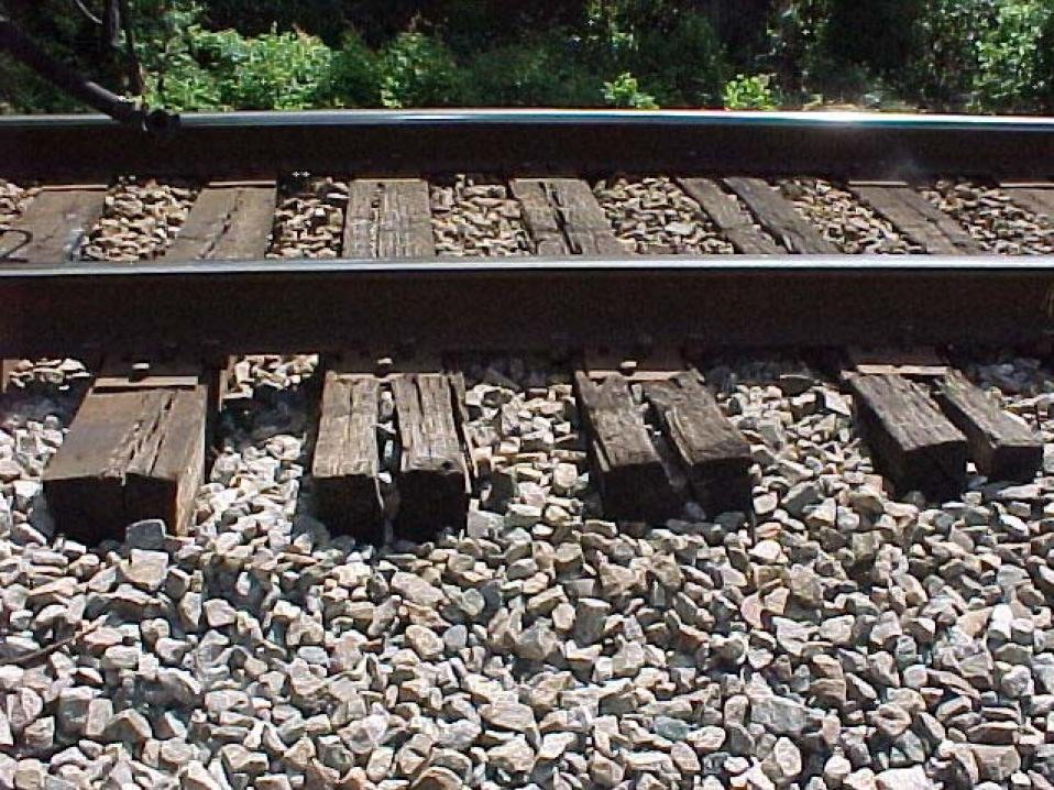
Ballast sloping off. the ends of the ties
