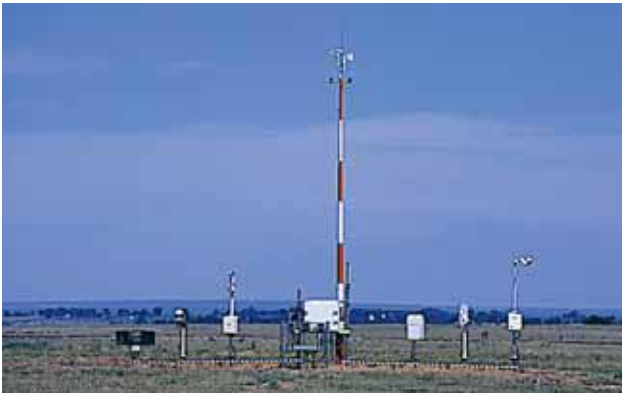
Figure 2-12. ASOS Station Installation.
