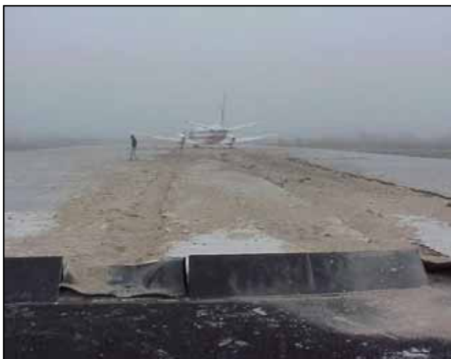
Aircraft stopped by EMAS at JFK
