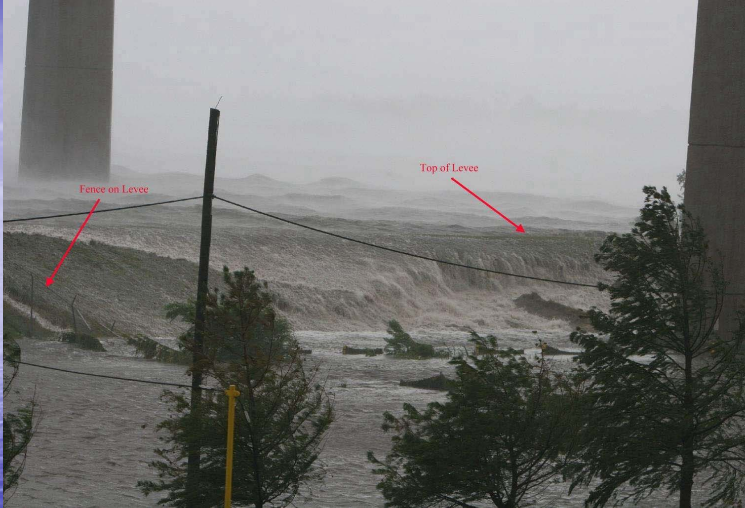
Hurricane Katrina - A massive wave crashes over a floodwall at the Paris Road bridge near Michoud's Entergy plant in New Orleans near I-510
