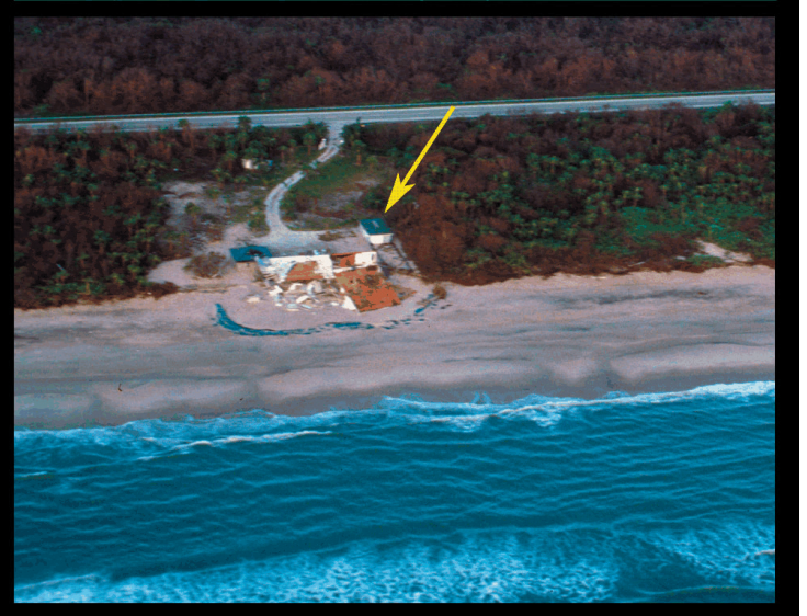
Hurricane Frances before and after photo of an oceanfront house destroyed by waves and erosion on North Hutchinson Island, FL. Note how the vegetation/dune line is now more landward than before the storm, indicating erosion. Also note the remains of a protective seawall on the beach.
