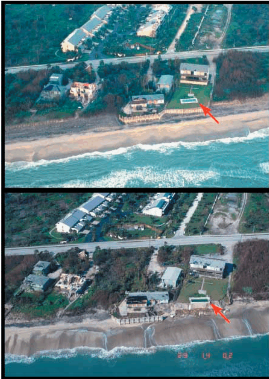
Dune erosion and seawall failure, Melbourne Shores, FL: The upper photo is post-Frances and the bottom photo is post-Jeanne. The seawall on the right survived Hurricane Frances, but failed during Jeanne. Note the extreme dune erosion where the front face of the dune retreated landward to the pool.
