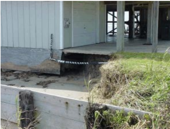
Figure 1: Beach Erosion in Bermuda Beach. (Photo courtesy of the Texas General Land Office)
