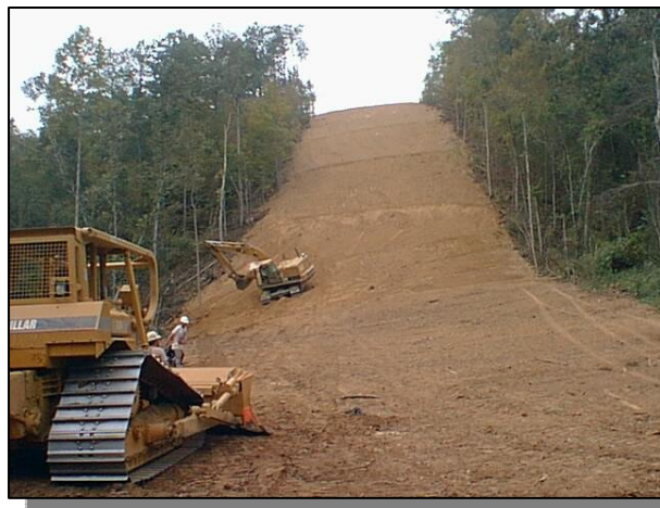
Figure 8. Typical Cross Slope Construction.
