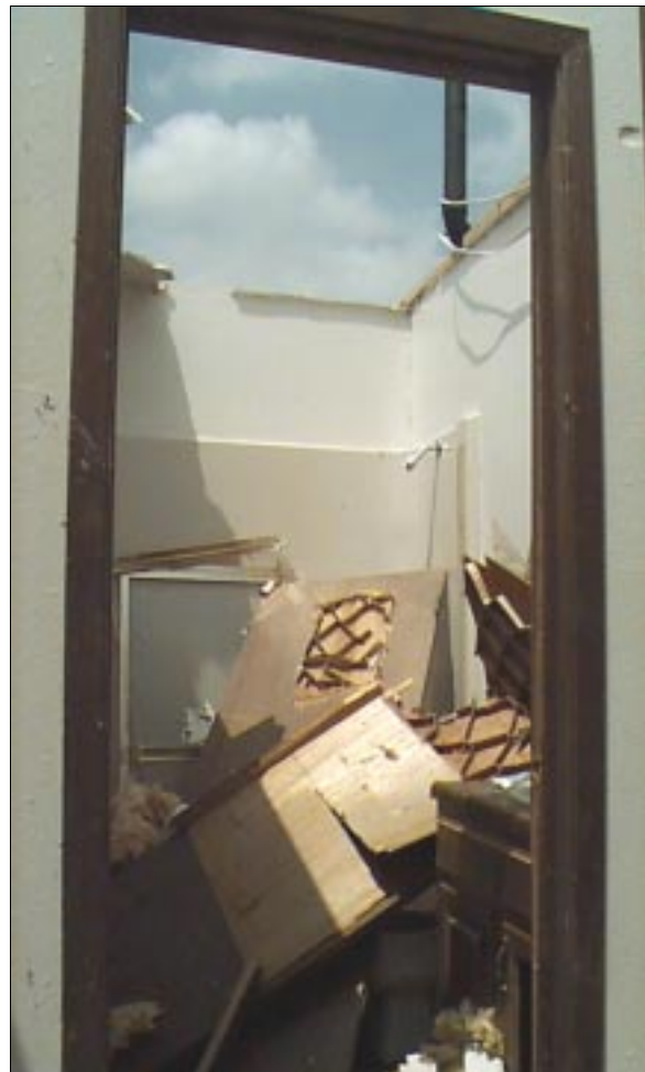
FIGURE 6-23: This house outside of Moore, Oklahoma, was affected by inflow winds associated with a severe tornado. The roof and ceiling were blown off of the interior bathroom of this house, the door was blown into the bathroom, and the tub was full of debris. This bathroom was not a safe refuge.
