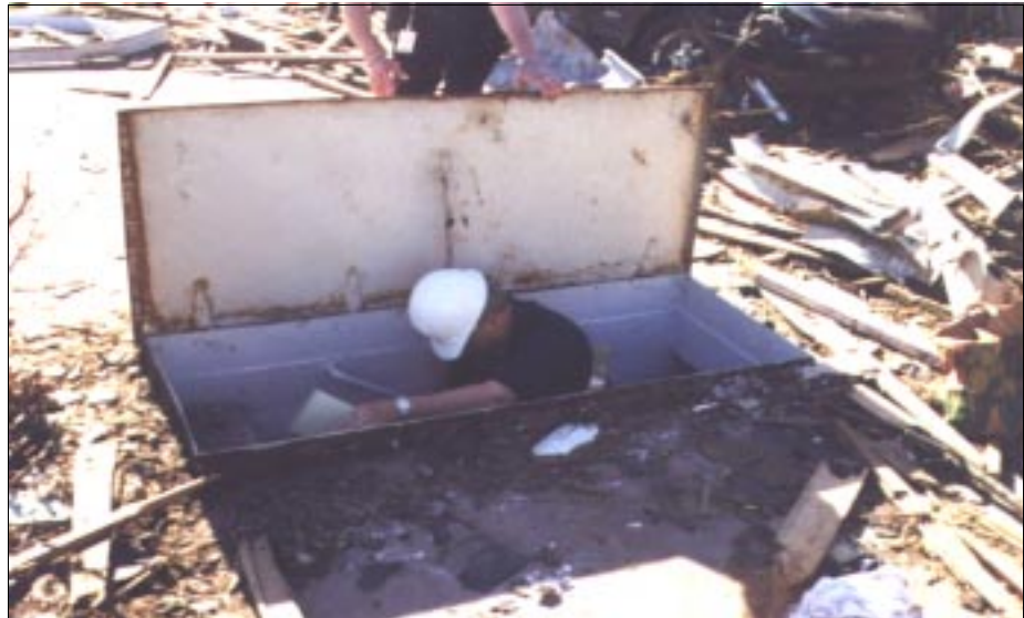
FIGURE 6-5: Del City storm cellar constructed of steel sheets with a concrete cover. This area was directly struck by the vortex of a violent tornado.
