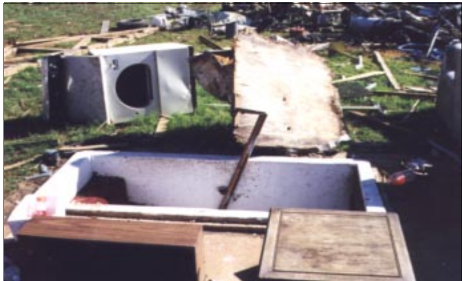
FIGURE 6-13: Failed wooden door at a below ground shelter in Oklahoma.
