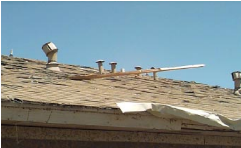
FIGURE 3-15: Windborne missile striking a house located in Moore, Oklahoma.
