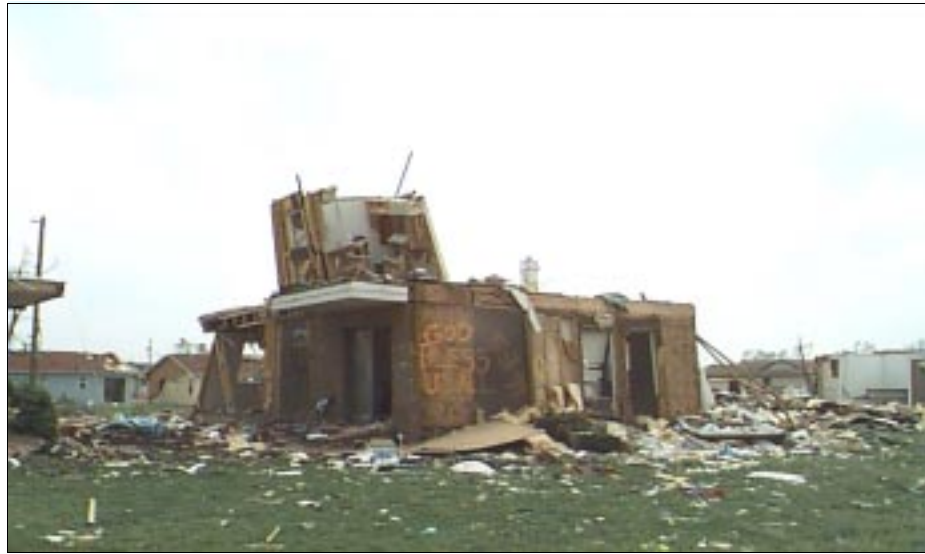
FIGURE 6-27: The second story of single and multi-family houses typically experienced far greater damage than the first story. This multi-family home in Wichita, Kansas, was affected by inflow winds of a severe tornado.
