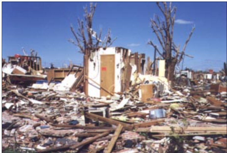
FIGURE 6-21: Remains of an interior room or core of a home in a Moore, Oklahoma, subdivision that was hit by a violent tornado.
