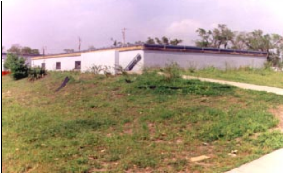
FIGURE 6-6: Community Shelter at a Wichita, Kansas, manufactured home park. While the park was directly hit by a severe tornado, the shelter was not within the damaged area.
