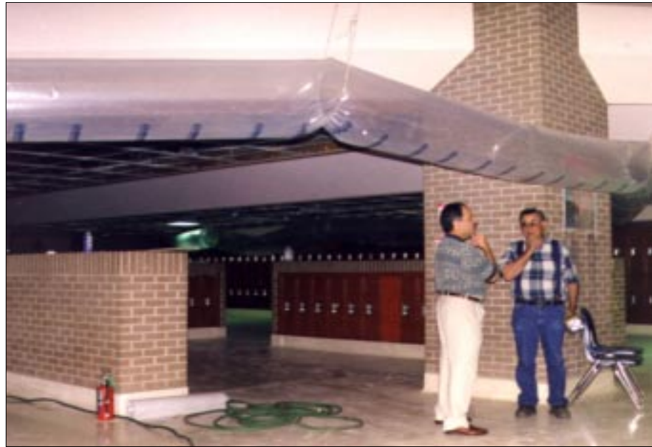
FIGURE 6-29: Westmoore High School, Moore, Oklahoma, central locker core - a designated place of refuge.
