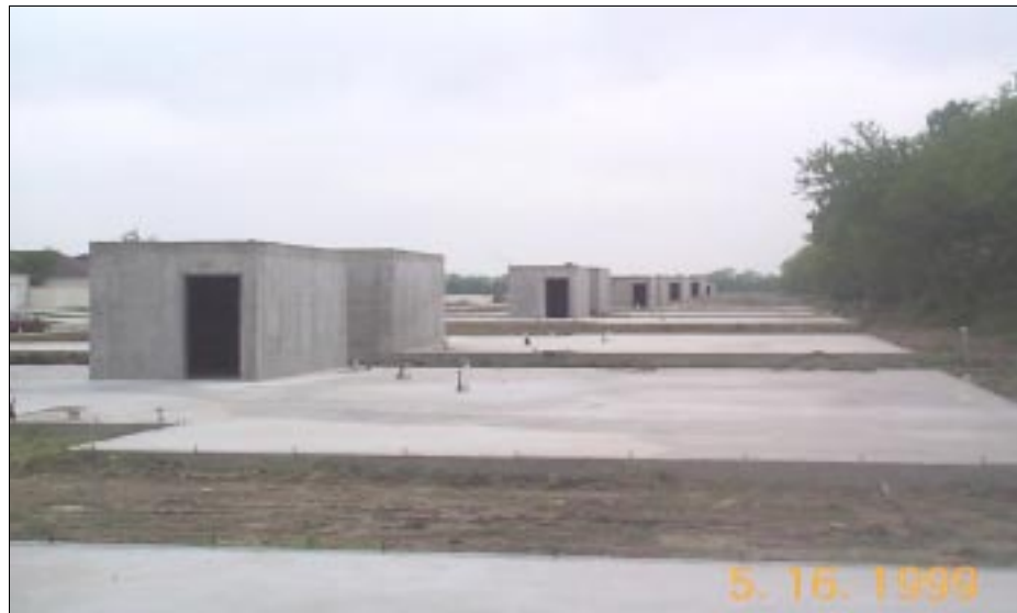
FIGURE 6-7: Above ground in-residence shelters under construction in Wichita, Kansas.
