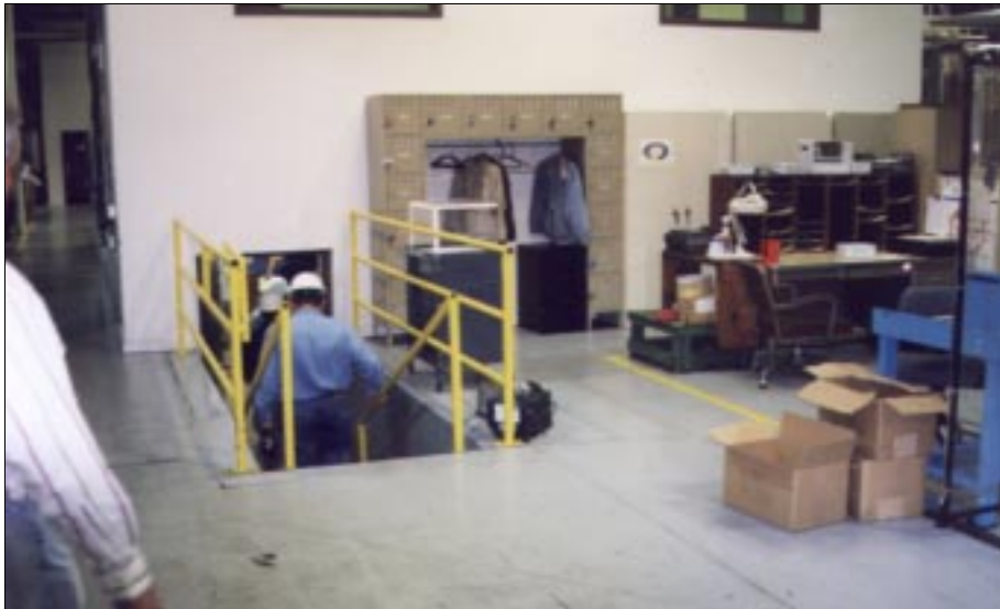
FIGURE 6-8: Entrance to the plastics manufacturing plant group shelter in Haysville, Kansas.
