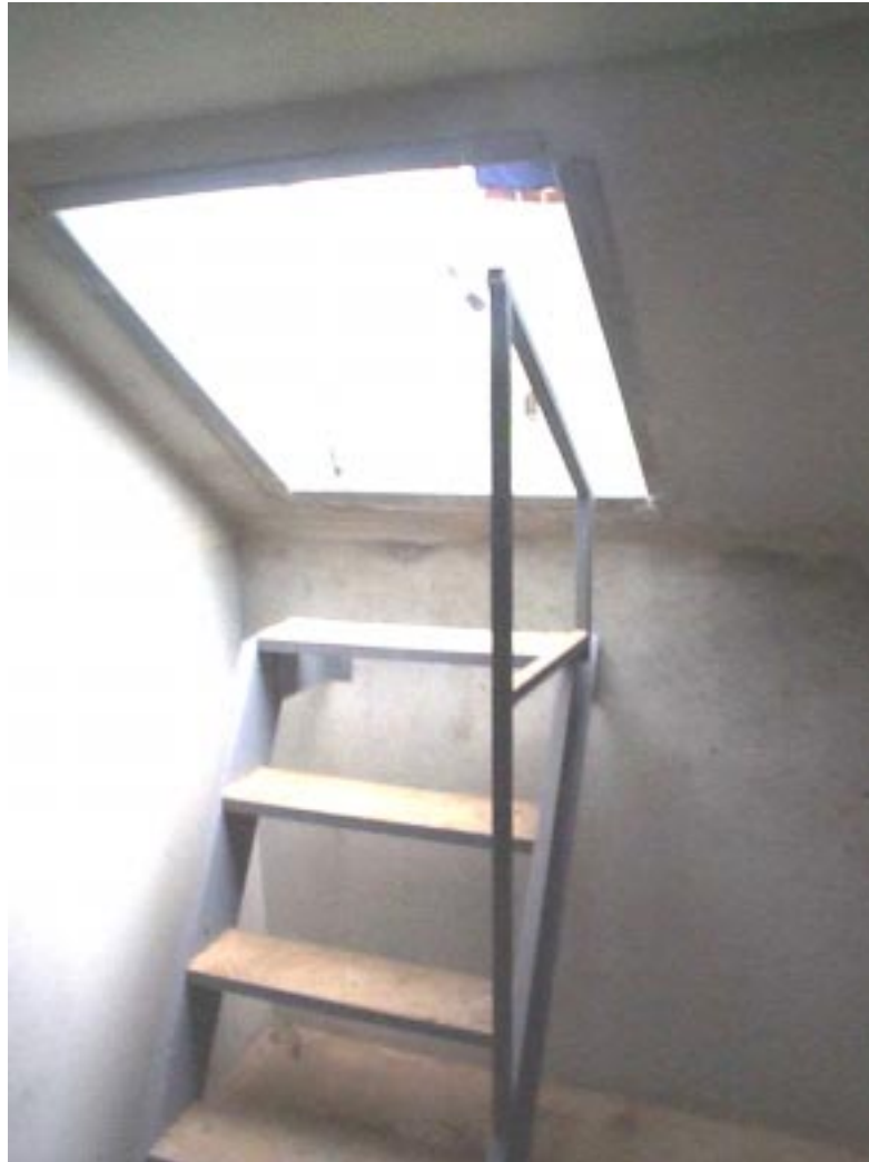
FIGURE 6-17: Stairway access to group shelter at manufactured home rental development, Wichita, Kansas. This development was not affected by any of the tornadoes that struck on May 3, 1999.
