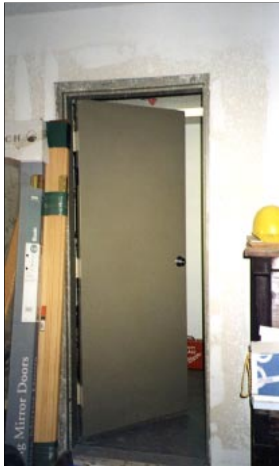
FIGURE 6-3: Entrance to the ICF shelter in Bridge Creek, Oklahoma. This residence and shelter were on periphery of the inflow winds of a violent tornado, and damage was limited to light missile impacts.
