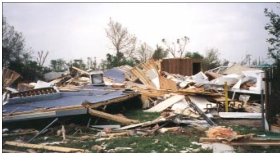
FIGURE 6-28: Damaged and destroyed manufactured homes in Wichita, Kansas, that were in the direct path of a severe tornado.
