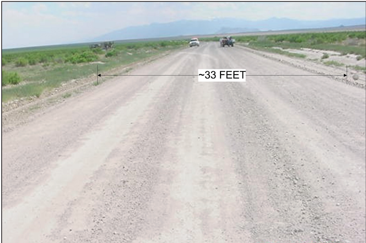
Photo 1. Incident Site Photo courtesy of State forestry department
