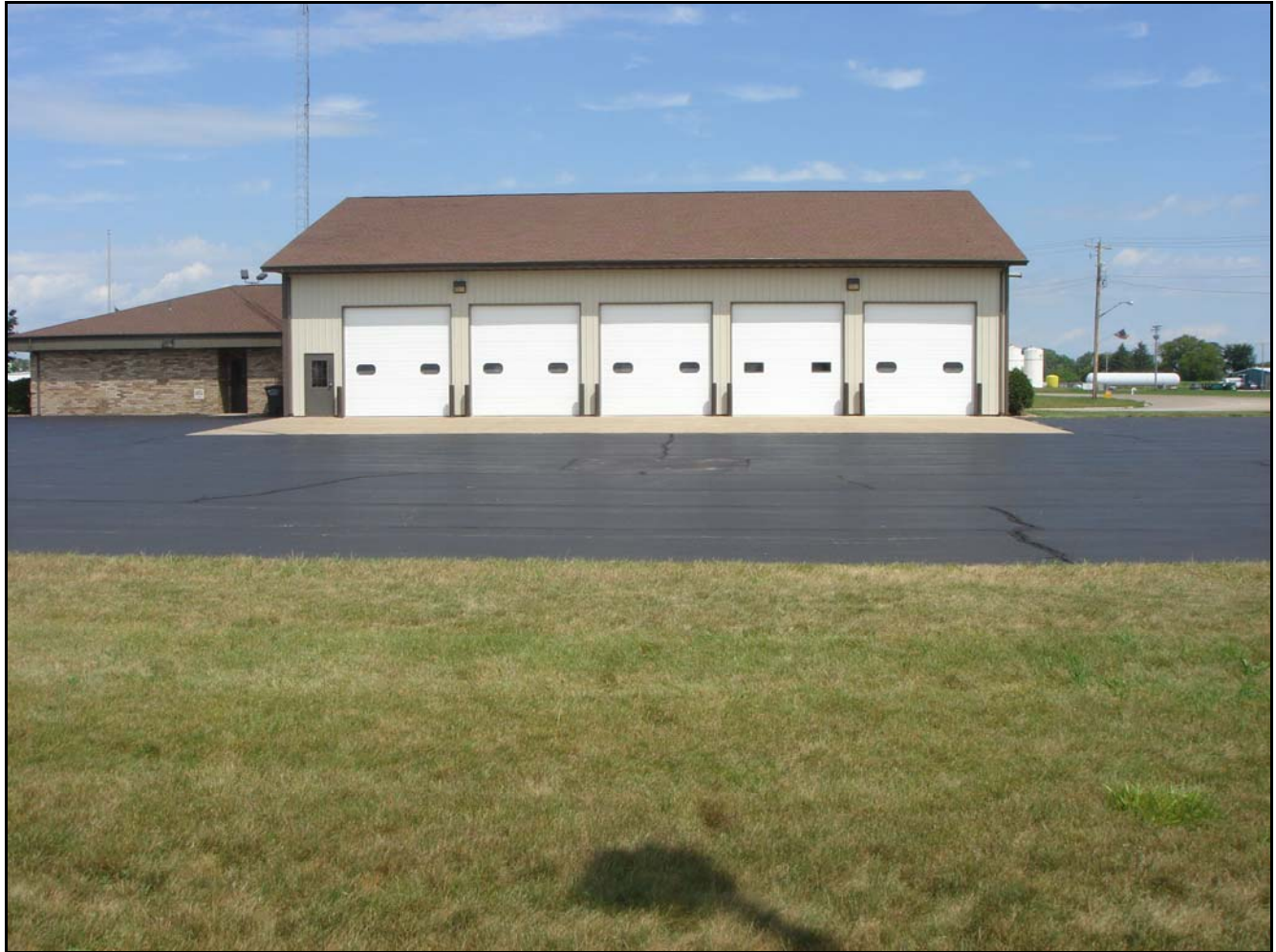
Photo 7. Parking available at rear of station where incident occurred. (NIOSH Photo)
