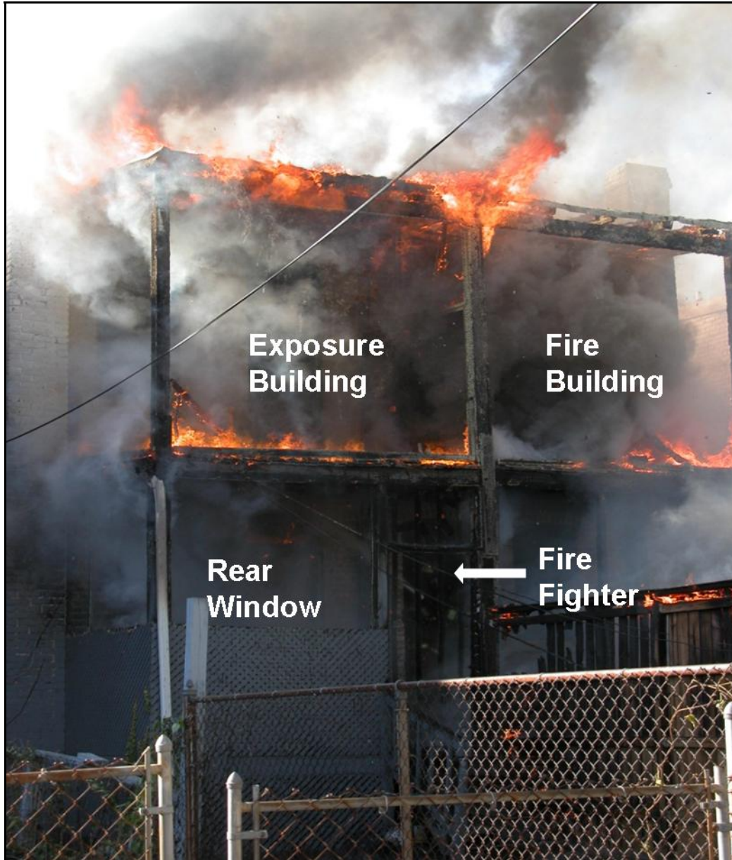
Photo 1. Fire fighter attacking fire through a rear window from the back porch area on side-C of exposure building at approximately 1528 hours; illustrates fire extending inward. ( Photograph courtesy of the fire department. )
