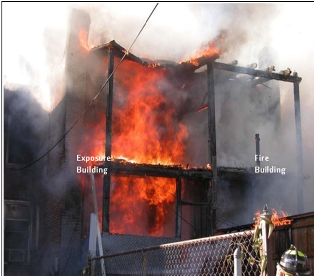
Photo 3. Fire travels up interior stairwell and up exterior back wall to second floor of exposure building at approximately 1530 hours and fire fighters are burned. (Photograph courtesy of the fire department.)
