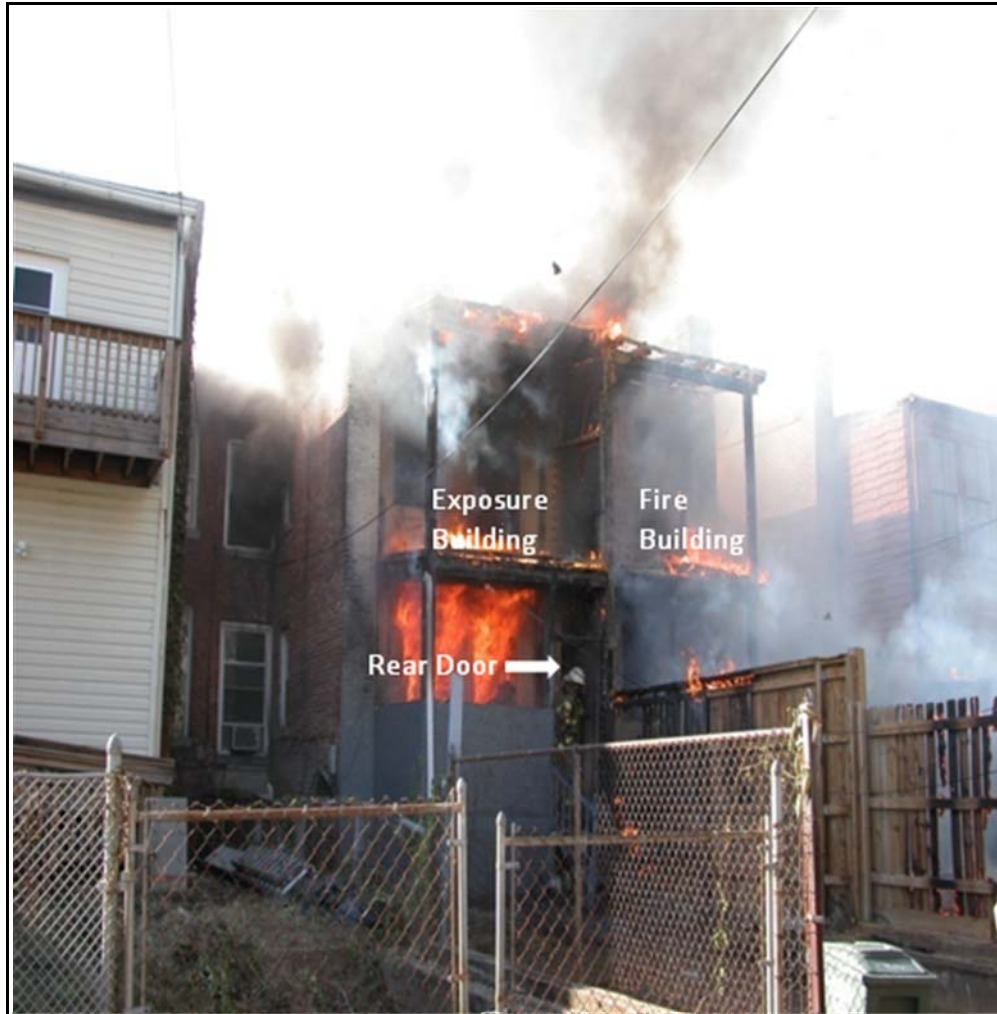
Photo 2. Rear door of exposure building (side-C) is opened at approximately 1529 hours and conditions on first floor and second floors deteriorate. (Photograph courtesy of the fire department.)
