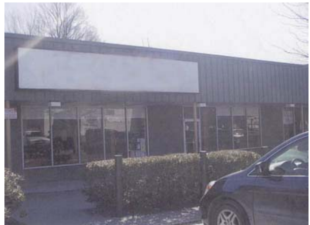
Photograph 1. Restaurant located in a strip mall.
