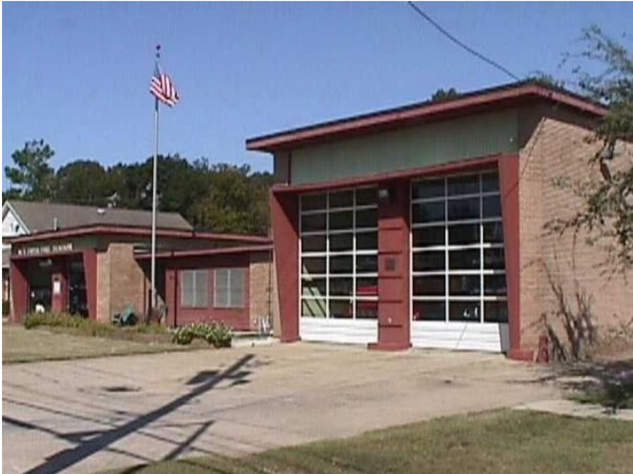
Photo 2. Station's Driveway Apron
