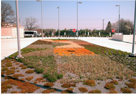
Top: Green roof atop Bldg. 66, the new NIH Gateway Center
