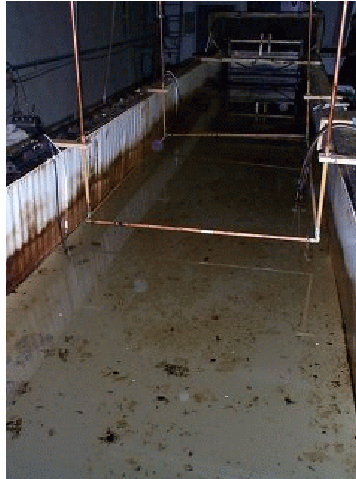
Figure 2: Air Bubble Curtain Piping
