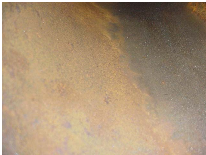
Line 25 – Internal Pipe Photos
