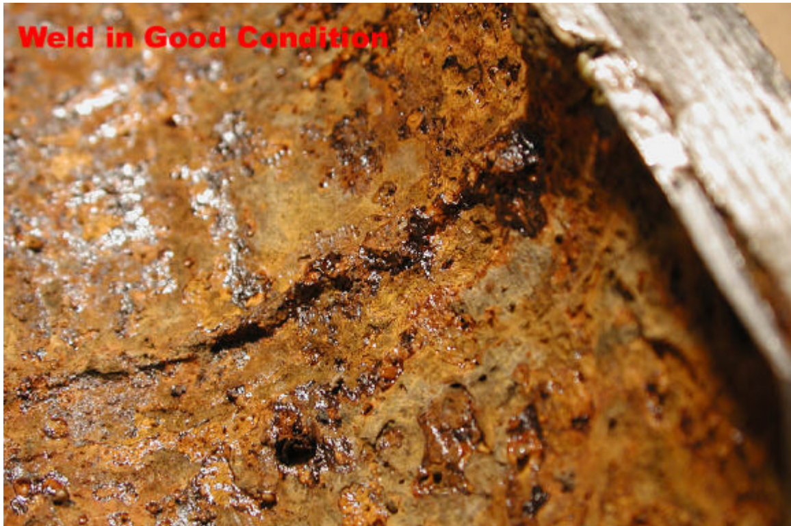
Photo #27 - Sample Photo – 2826 Pipeline to Tubeturn Weld
