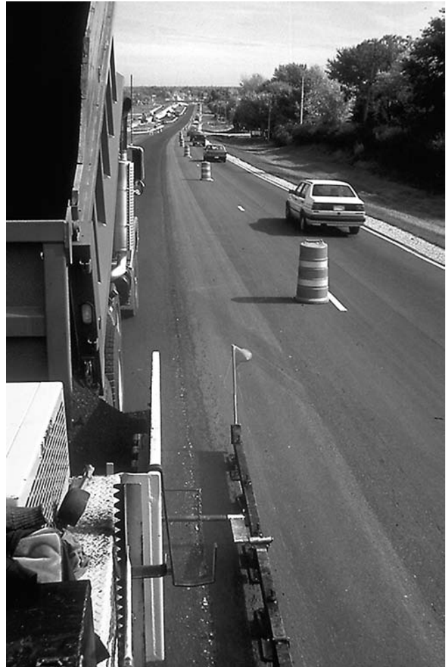
FIGURE 16-5 Floating-beam mobile reference.
