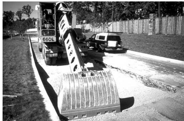
FIGURE 14-2 Removal of existing pavement prior to patching.
