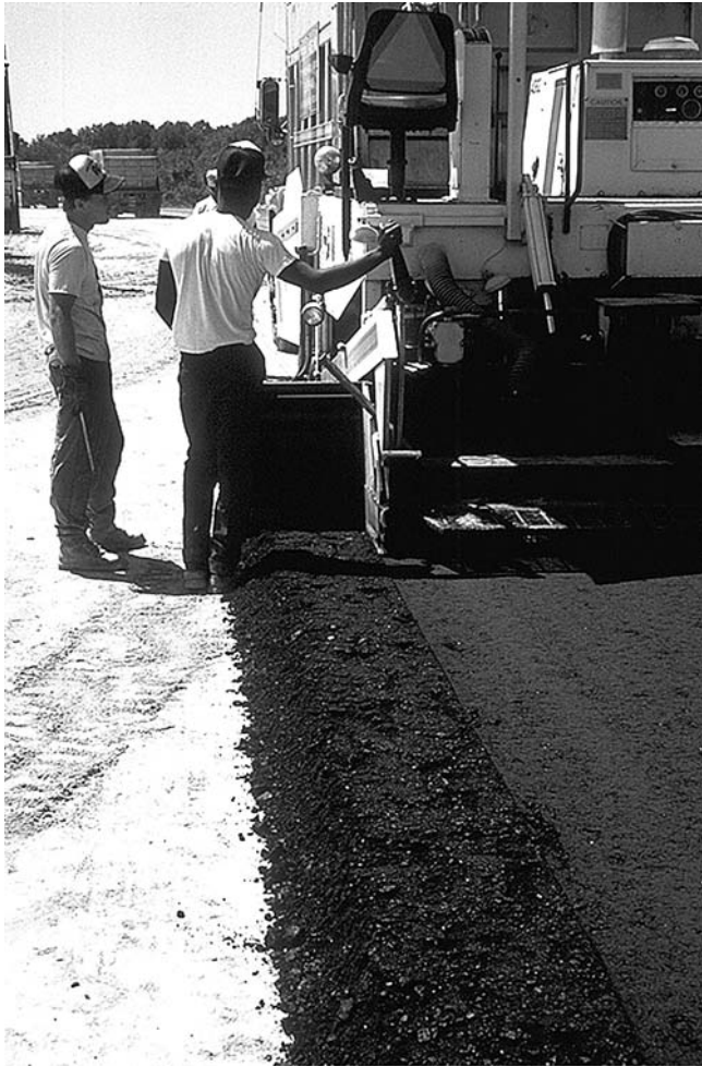
FIGURE 15-19 Difference in texture under strike-off extension.
