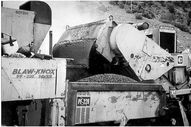
FIGURE 15-3 Windrow elevator.
