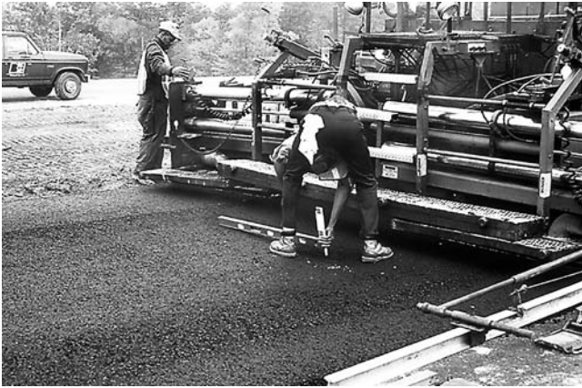
FIGURE 16-11 Checking slope of mat surface behind paver.
