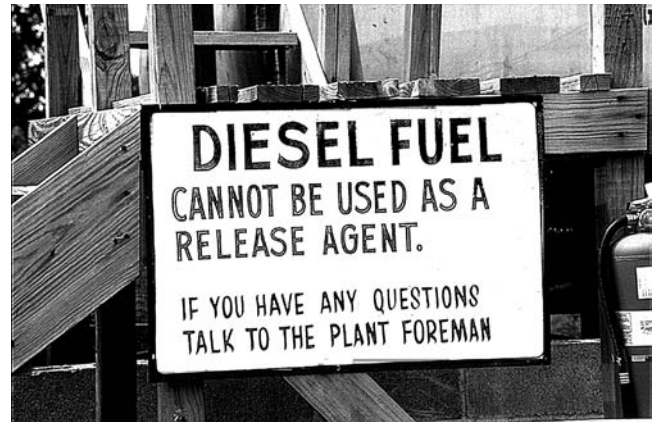
FIGURE 13-6 Diesel fuel is an unacceptable release agent.
