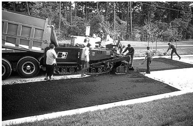
FIGURE 14-1 Patches placed with paving machine.
