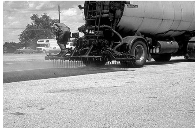
FIGURE 14-7 Distributor applying tack coat.
