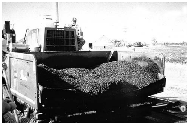
FIGURE 15-2 Loaded HMA paver hopper.
