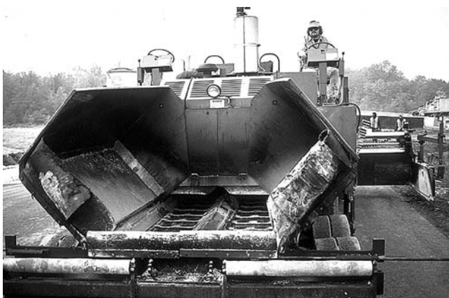
FIGURE 15-4 HMA paver with wings lifted.
