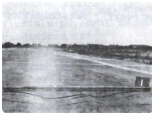
SURFACE OF OVERLAY
