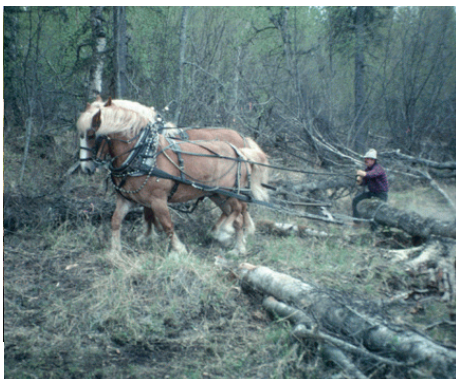
Using draft horses to place logs for streambank restoration.
