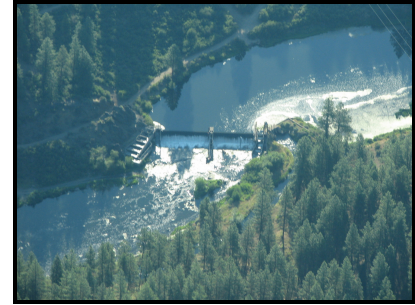
The Chiloquin Dam impedes fish movement on the Sprague River. It will be removed in 2008.
