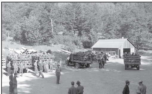
Camp Rand, May 27, 1935 Crews Loaded into Trucks Ready to Leave for Work
