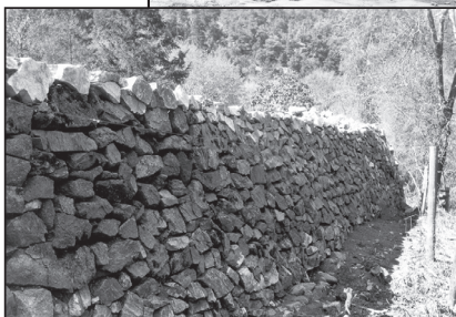
Retaining Wall Built by CCC, April 9, 1936
