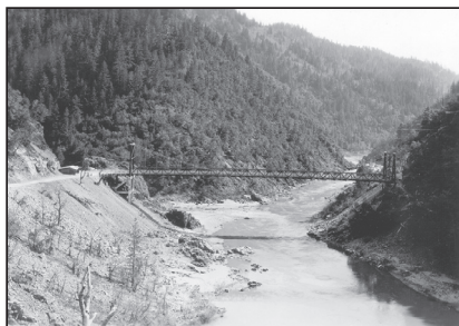
Grave Creek Suspension Bridge Built by CCC, April 9, 1936
