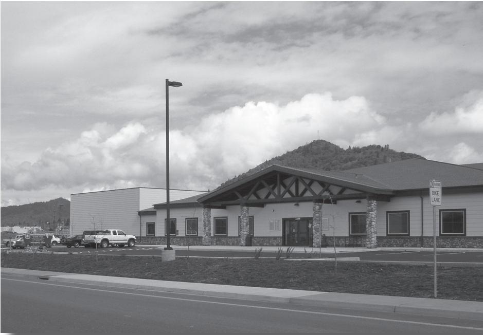
Opened in the fall of 2005, the Grants Pass Interagency Office is the home to BLM Medford District's Grants Pass and Glendale Resource Areas as well as part of the Rogue-Siskiyou National Forest.
