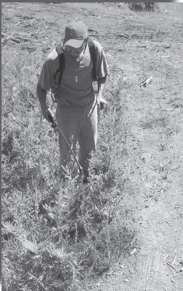
A contractor treats roadside weeds by handspraying. The herbicide is combined with a blue dye which will show the contractor where he has sprayed and will allow the contract administrator to see that the herbicide is disposed of properly.
