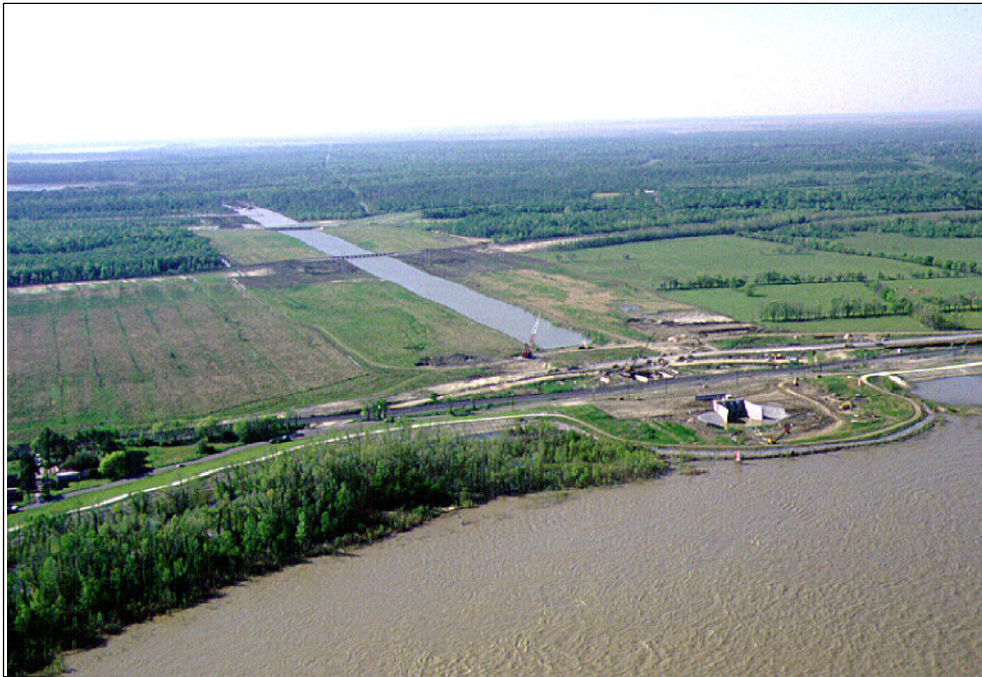
The Davis Pond structure, looking south toward Lake Salvador and the Barataria Basin. River water, up to 80,000 gallons per second, will be diverted to the outflow channel, eventually into the 9,300-acre ponding area and then toward the Gulf of Mexico. The total project area is 10,084 acres.
