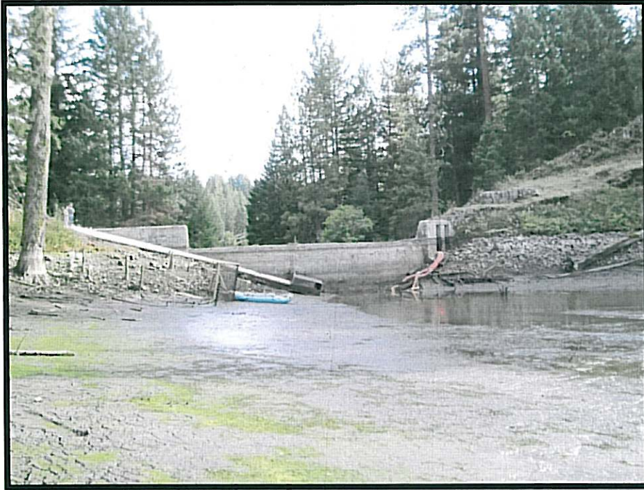
PHOTO 3 – UPSTREAM FACE OF DAM
