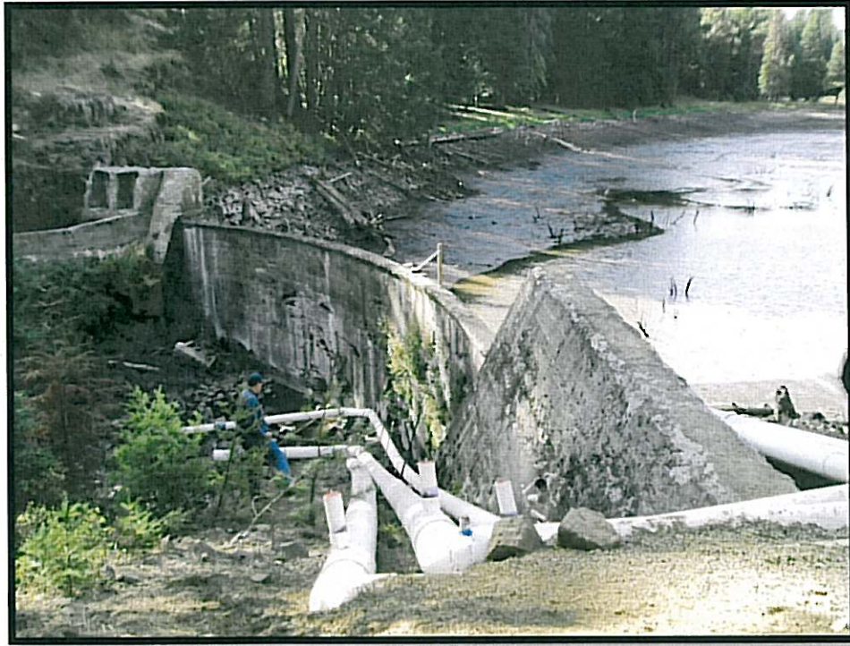
PHOTO 1 - DOWNSTREAM FACE OF DAM
