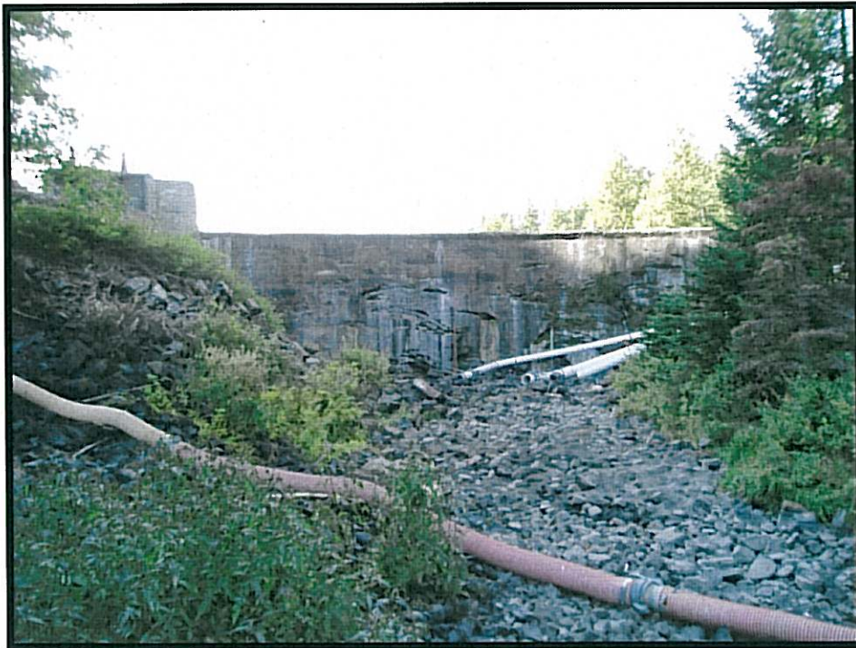
PHOTO 2 - DOWNSTREAM FACE OF DAM
