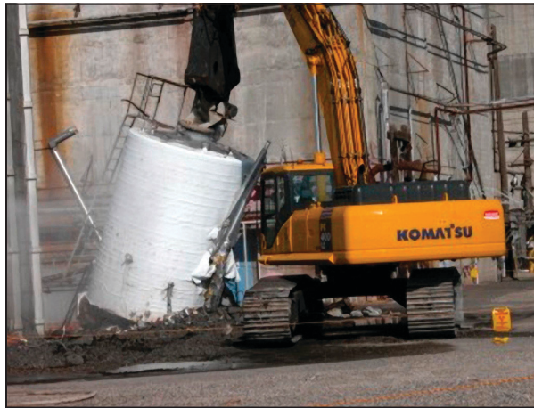
A Mechanical Shear Demolishes an Excess Storage Tank at Hanford
