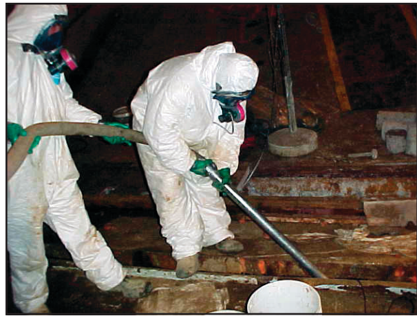
Brookhaven workers remove contaminated soil
