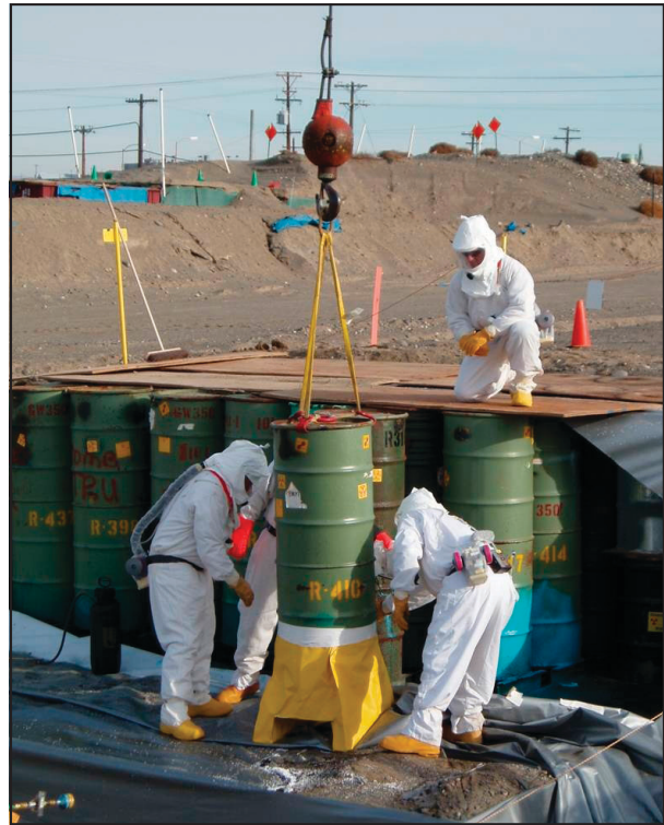
Retrieving Waste Drums at Hanford
