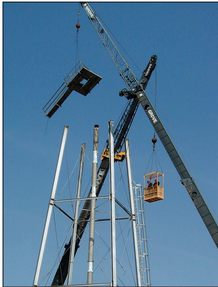
Dismantling a water tower at Hanford
