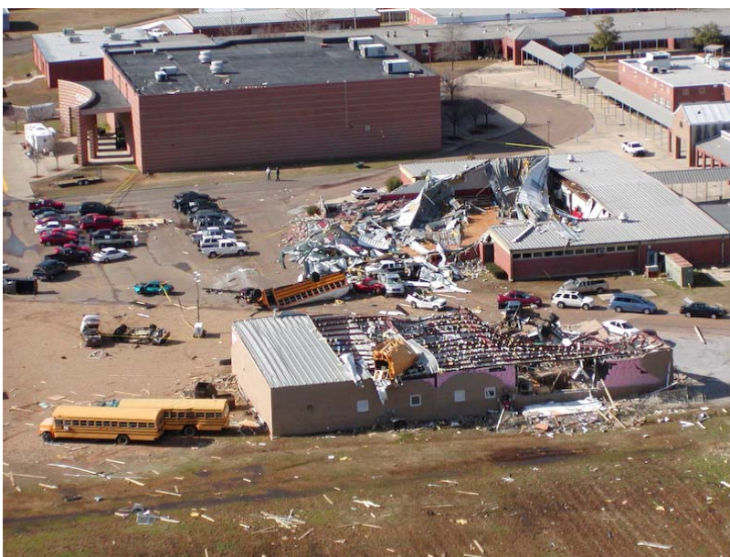
The image above shows an aerial view of the tornado damage. The building closest to the bottom is what remains of the Vocational Tech building. The damaged building in the middle of the picture is what remains of the gym. The remainder of the school complex had very little damage. The damage at this location was rated EF3 with estimated maximum winds of 155 mph.
