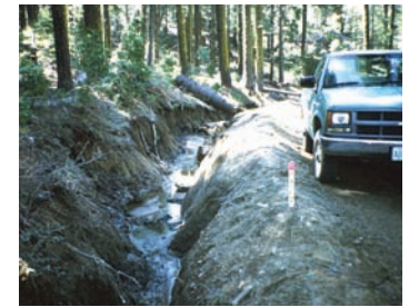
Hundreds of miles of Level 2 roads do not receive needed annual maintenance
