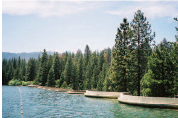
The Hume Lake Dam was the first multiple arch concrete dam constructed in the country.
