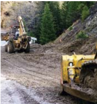
Road improvements will greatly enhance safety and access in many areas.
