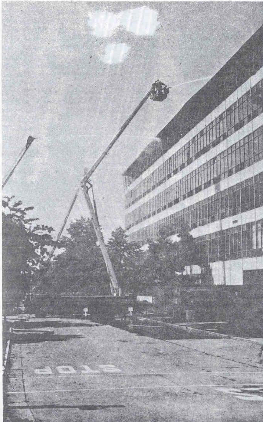
Fire department snorkels fighting the fire. Note the outward deflection of the sixth floor curtain wall.
