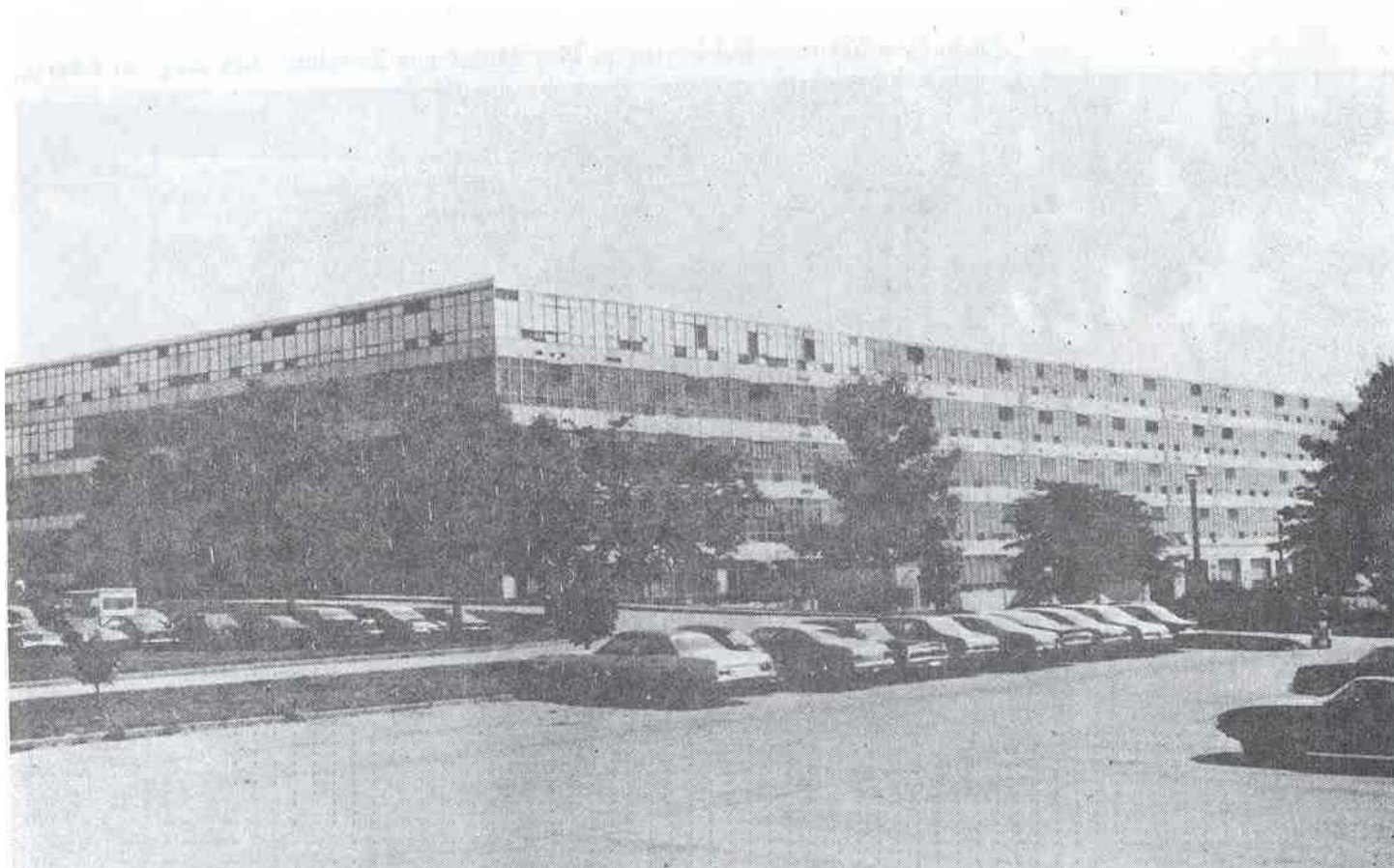
National Personnel Records Center after removal of the fire-damaged sixth floor. (Photograph by Larry Brock.)
