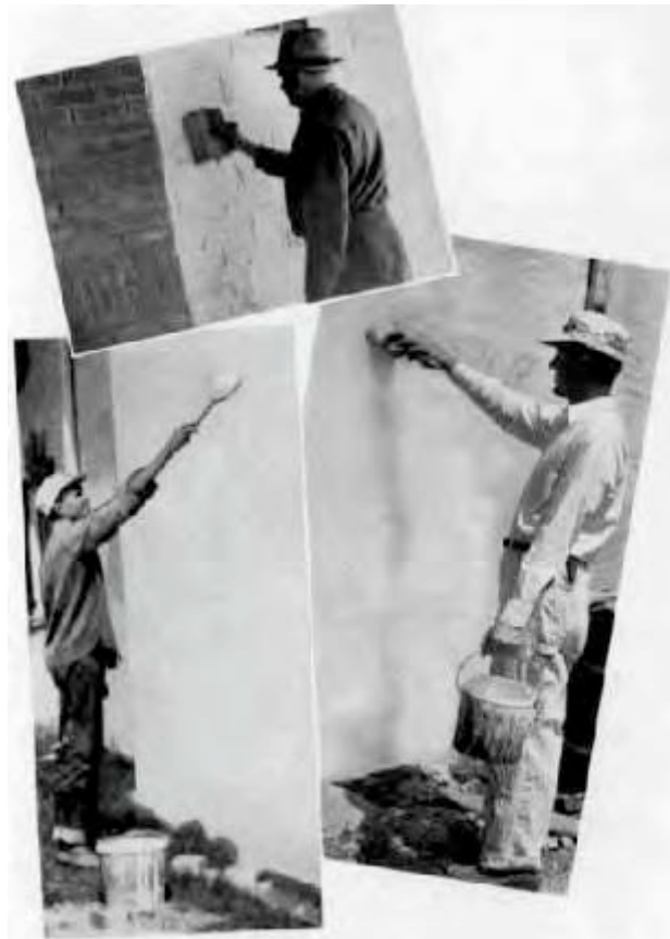
Whitewash is easily applied. The materials required are inexpensive, yet a good finish can be obtained if the surface is properly prepared and the whitewash applied thin.
