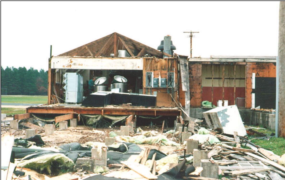
Figure 2. Mess hall under deconstruction.
