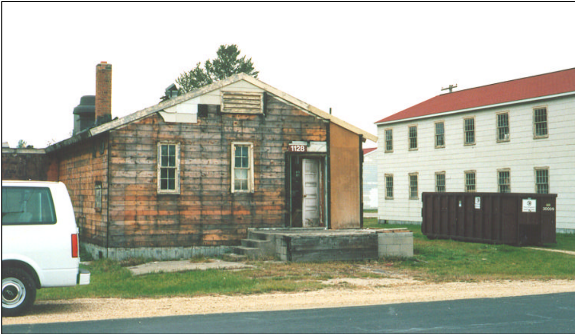
Figure 1. WWII building with siding removed.
