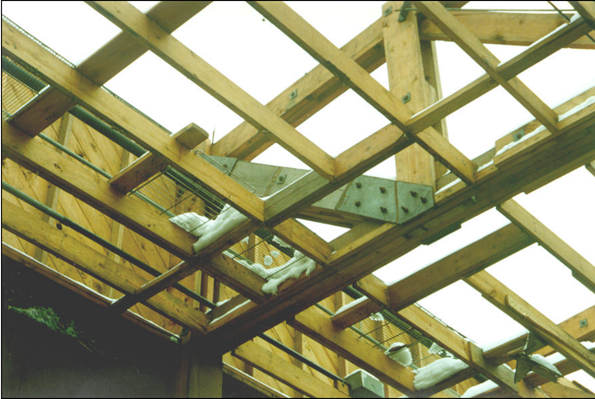
Figure 7. Theater building roof trusses.
