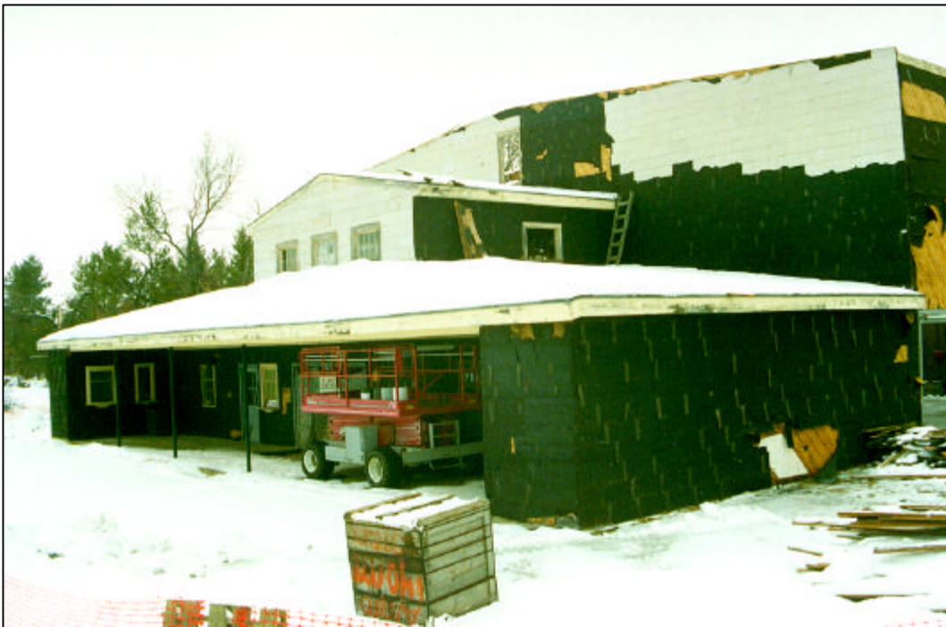
Figure 5. Exterior of WWII-era theater.
