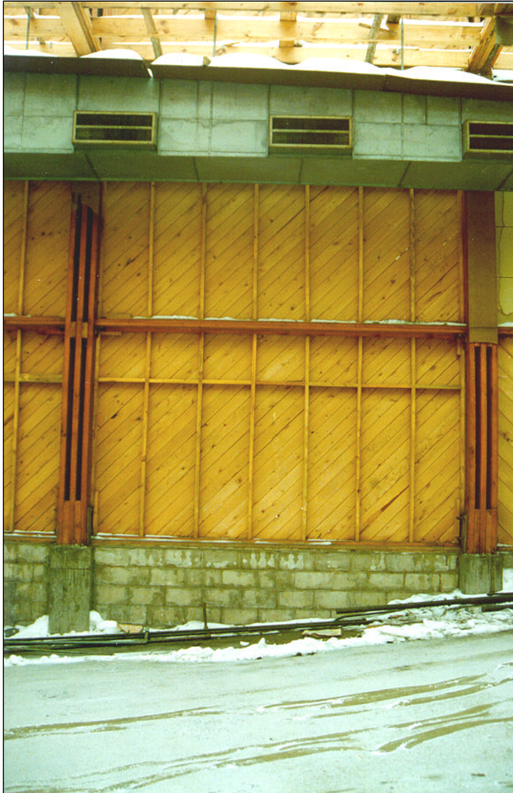
Figure 6. Interior wall of theater.
