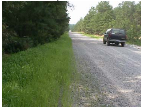
Harden and seed road shoulders on maneuver corridors and tank trails for stormwater harvesting and controlling erosion (Fort Bragg, NC).
