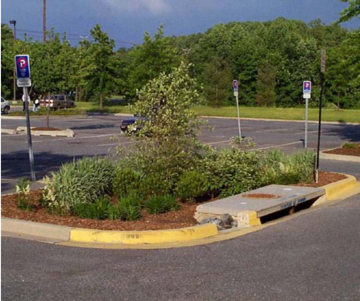
Figure A-9. A bioretention cell installed within an impervious area is one approach to stormwater management.
