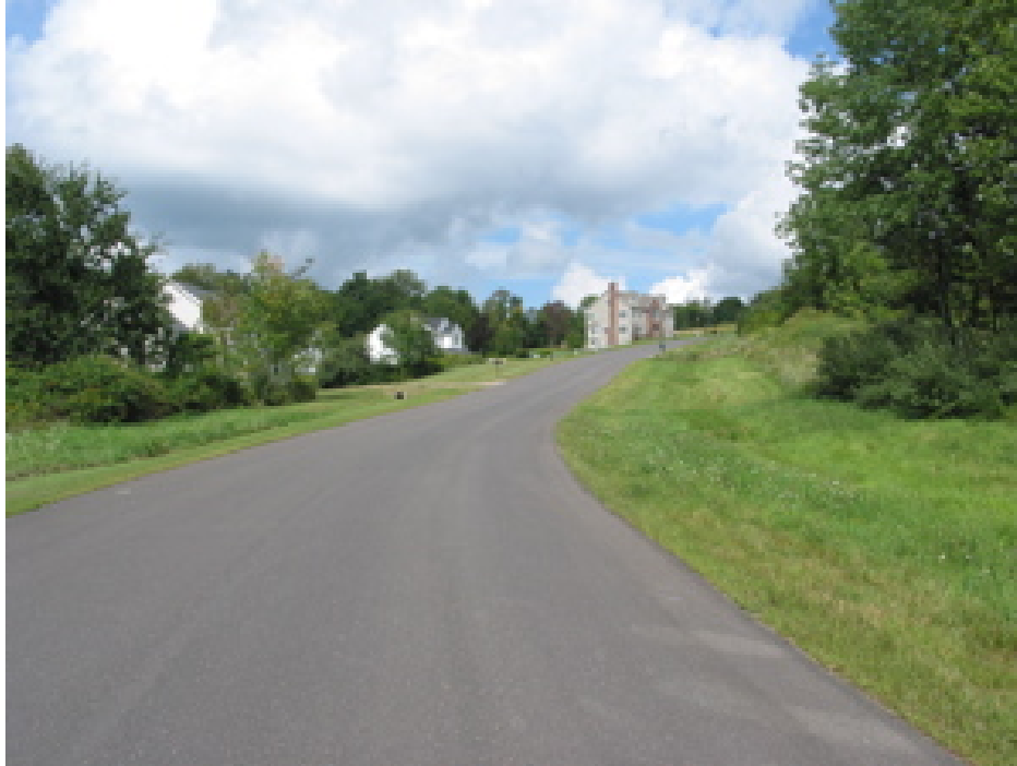
Figure A-6. Roads collect high concentrations of phosphorous, suspended solids, bacteria, and various metals, and generate high volumes of NPS pollution and concentrated runoff.
