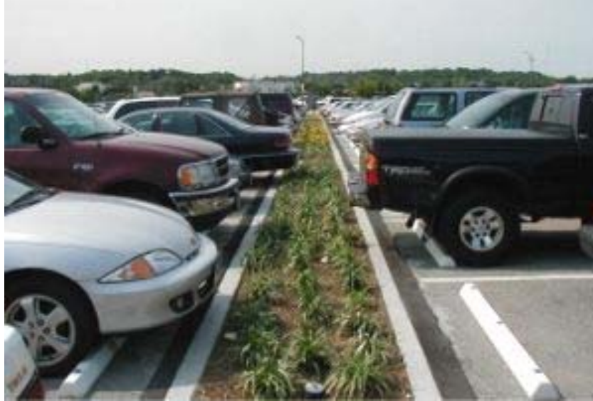
Figure A-4. Stormwater runoff is controlled close to the source by LID tools that promote water storage, infiltration, on-site water harvesting, and improved water quality.
