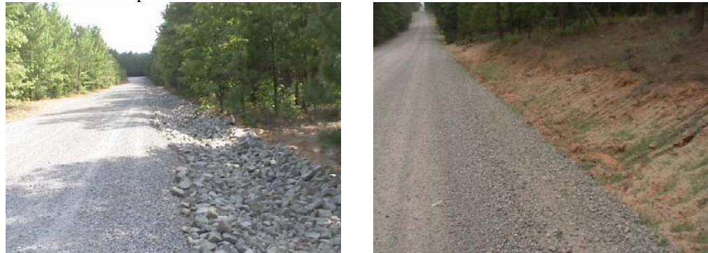
Example improved secondary roads at Fort Benning, GA.
