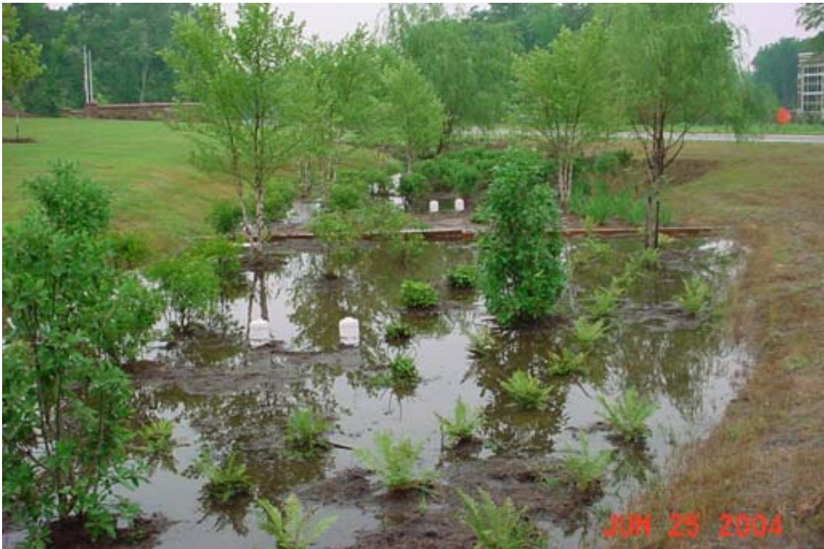
Figure A-7. James County Courthouse bioretention demonstration project taken during rainfall event (on-site stormwater runoff harvesting).
