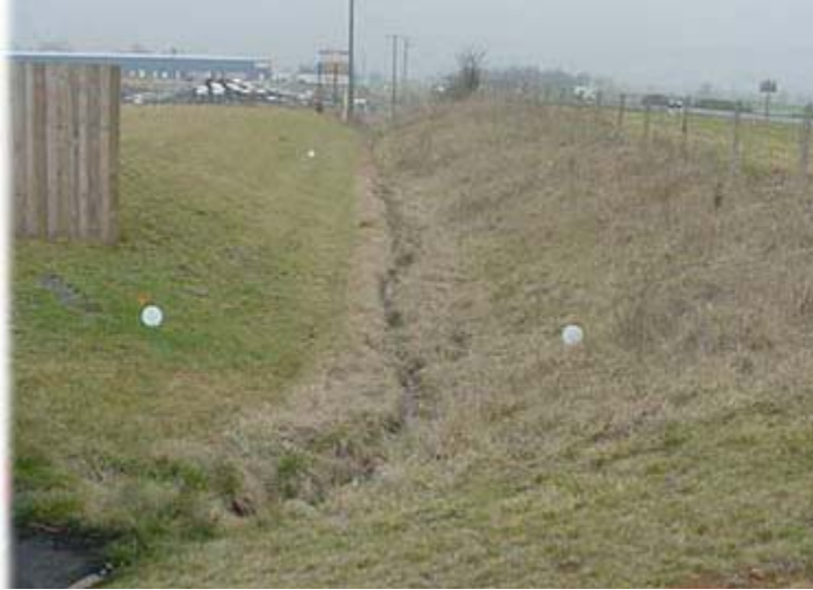
Figure A-10. The ditch where the rain garden was later constructed (Harrisonburg, VA).
