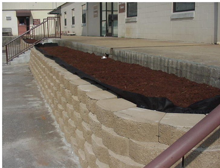
Newly constructed bioretention cell at Fort Bragg, NC.
