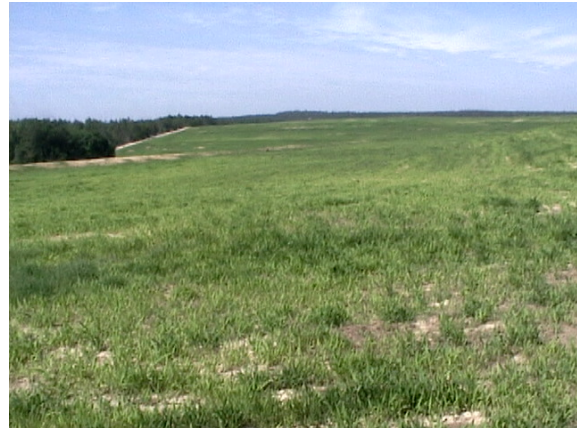
Figure A-5. Salerno Drop Zone, Fort Bragg, NC: Almost zero discharge is obtained by installing vegetated earth terraces that help retain, infiltrate, and store on-site storm runoff over large areas.
