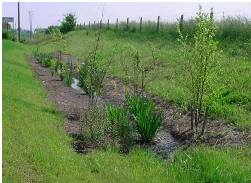
Figure A-11. Rain garden in June 2003, 14 months after construction (Harrisonburg, VA). When used as a LID IMP, this rain garden is an example of a bioswale.
