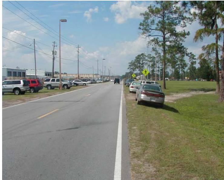
Figure A-18. Parking overflow and erosion at Fort Stewart, GA.
