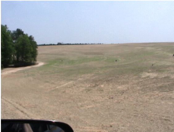
Figure A-5. Salerno Drop Zone, Fort Bragg, NC: Almost zero discharge is obtained by installing vegetated earth terraces that help retain, infiltrate, and store on-site storm runoff over large areas.
