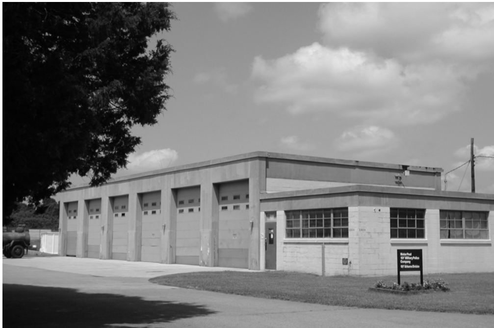
Figure C3. Motor pool facility.
