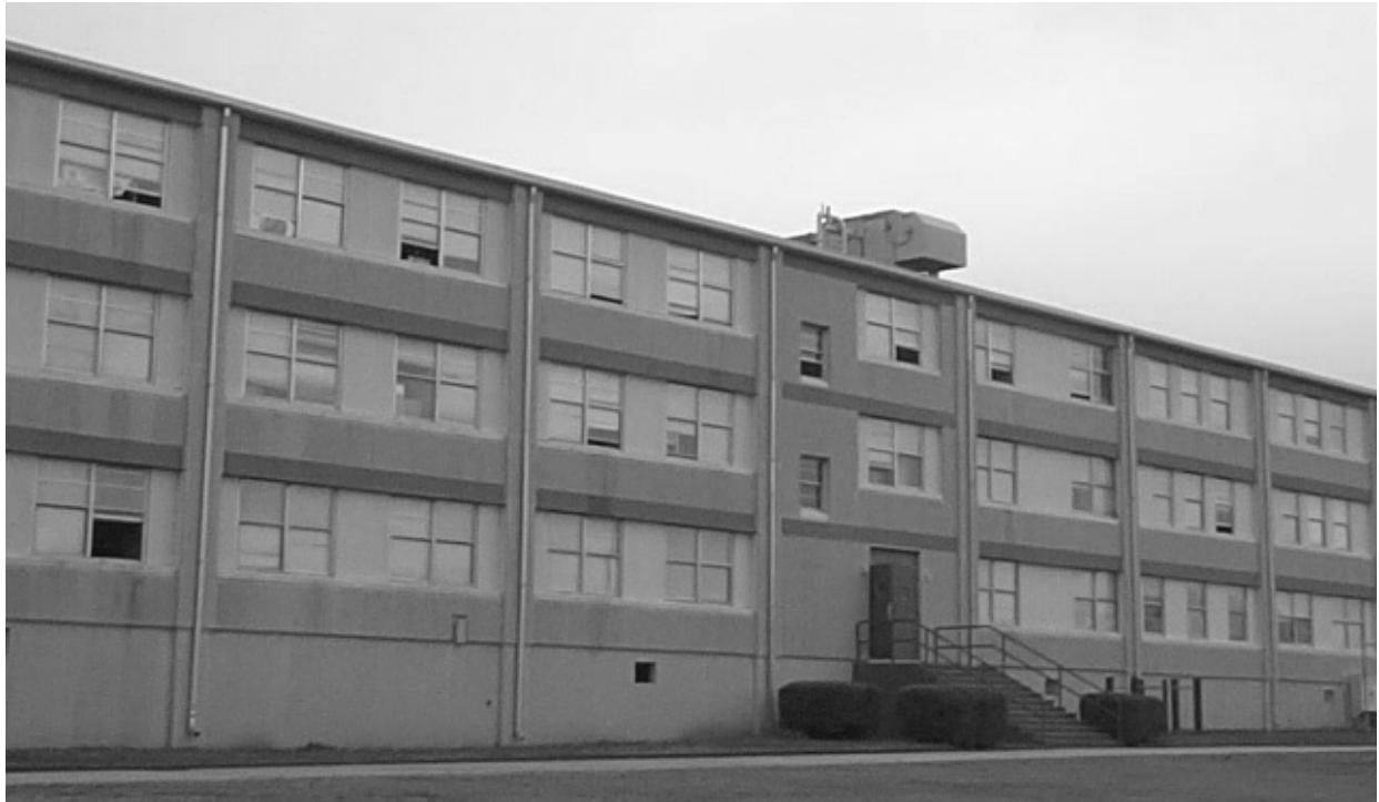
Figure C1. Exterior façade of Korean War-era barracks facility.
