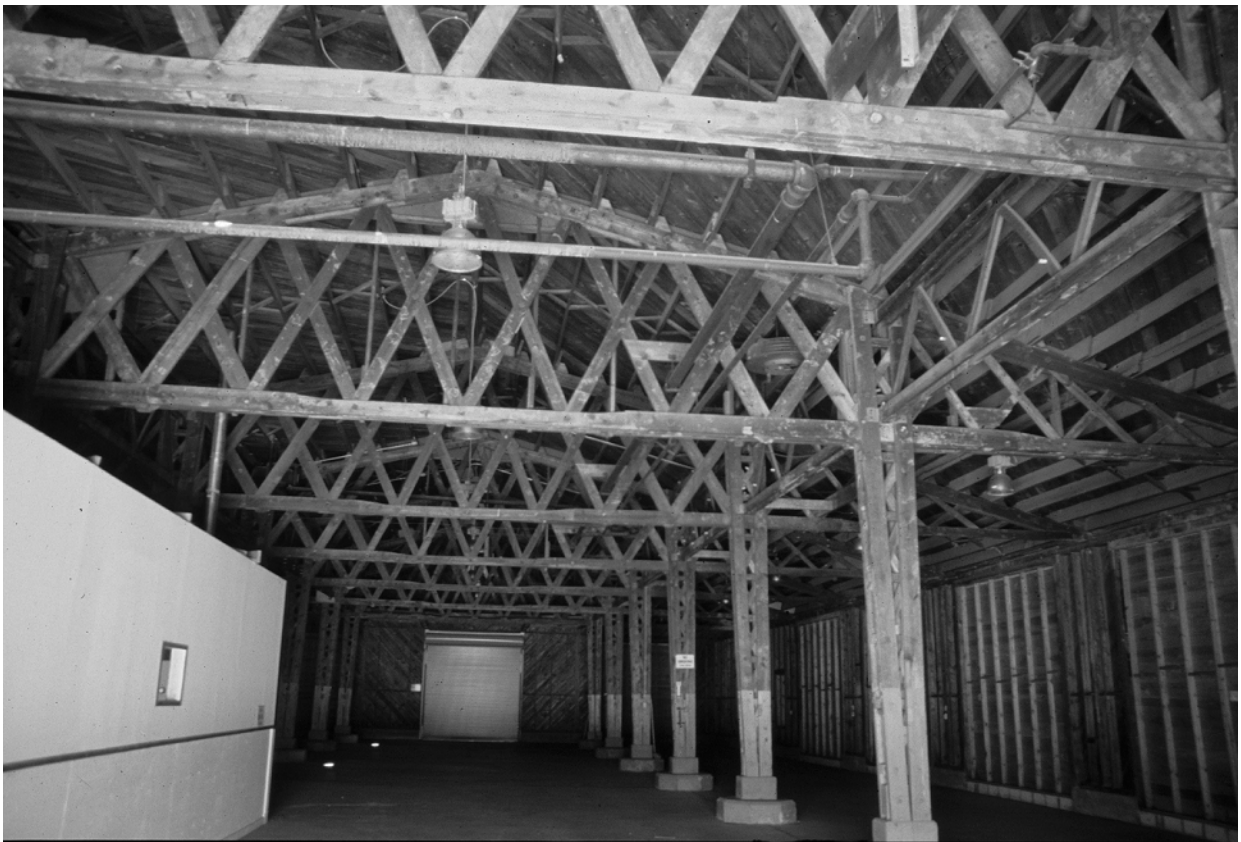
Figure B7. Interior of WWII-era heavy long-span structure.
