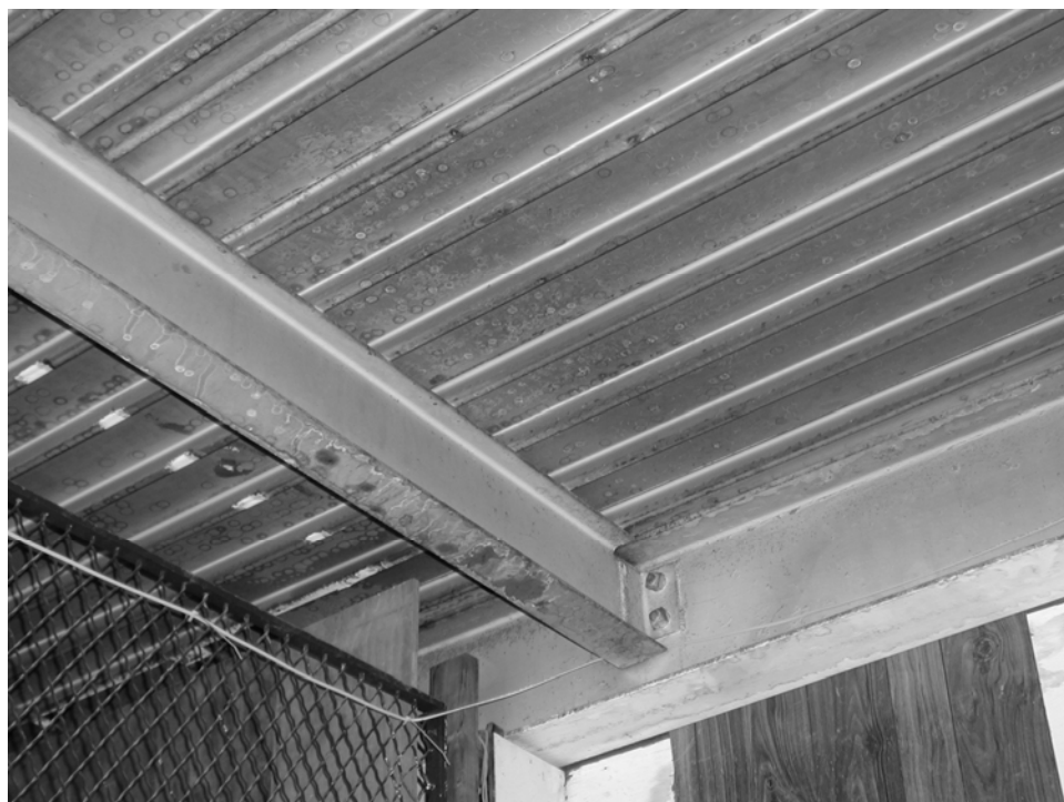
Figure C6. Motor pool facility roof construction
