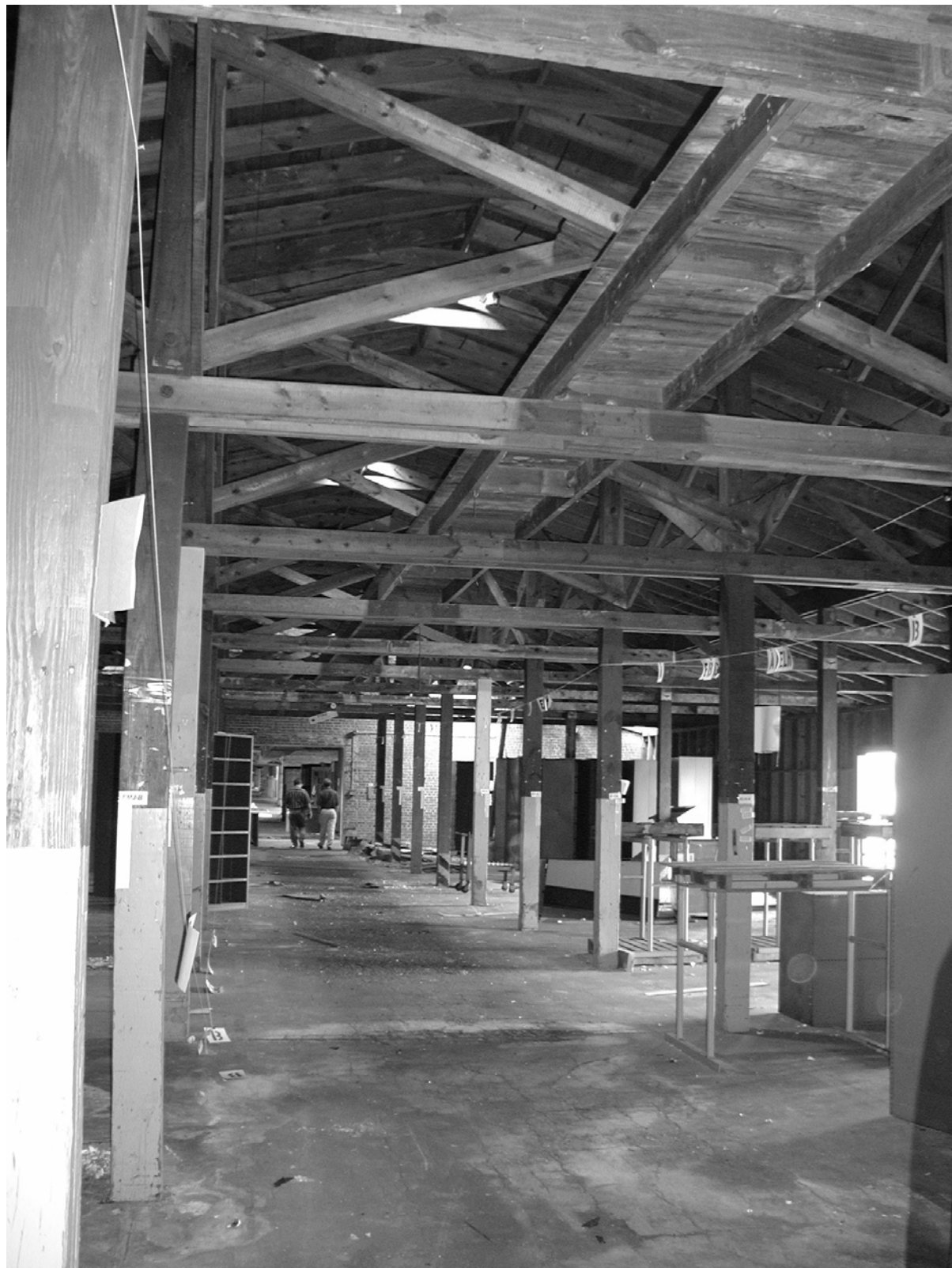
Figure B5. Interior of WWII-era light-frame wide structure.
