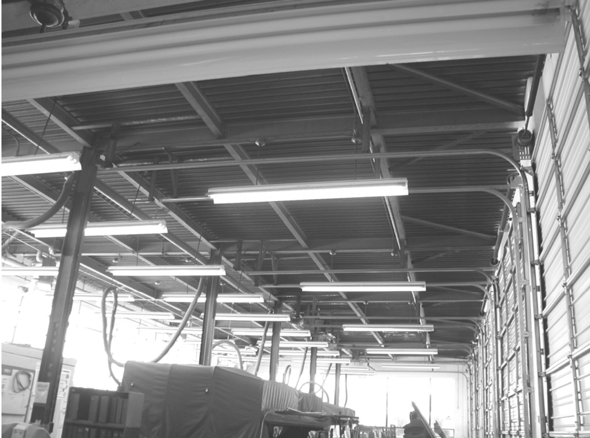
Figure C4. Motor pool facilities with interior steel columns.
