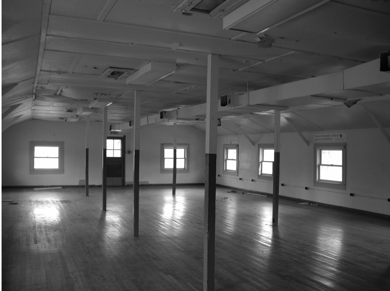
Figure B3. Interior of WWII-era light-frame two story building.
