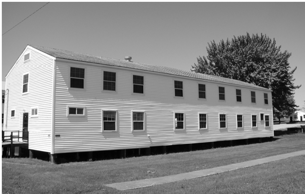
Figure B2. Exterior of WWII-era light-frame two story building.
