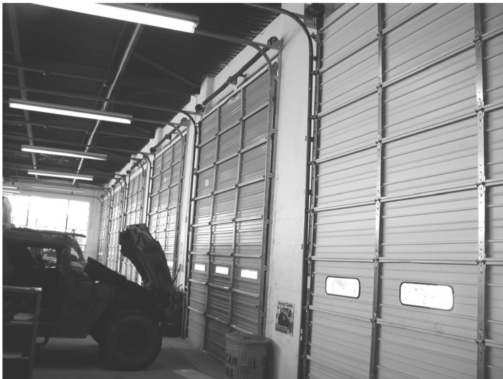
Figure C5. Motor pool facility with exterior perimeter concrete columns
