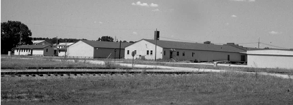
Figure B6. Exterior of WW-II era heavy long-span structures.
