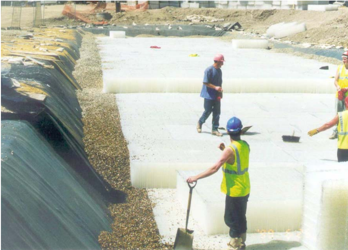
Figure B2. Stormcell® installed beneath the surface. (Used with permission.)
