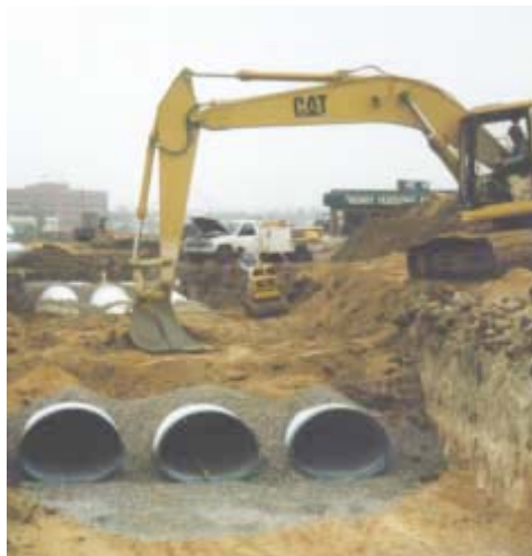
Figure A11. Installing corrugated metal pipes.
