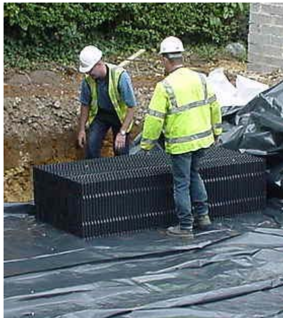
Figure B13. GEOlight is a thermoformed recycled PVC ultra-light honeycombed structure. (Used with permission.)
