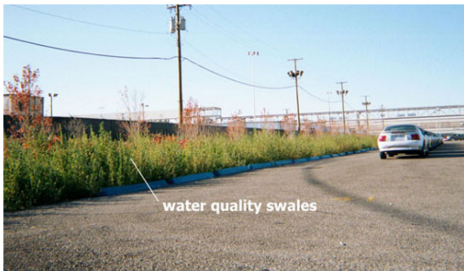
Figure A1. Vegetated water quality swales. (Used with permission.)
