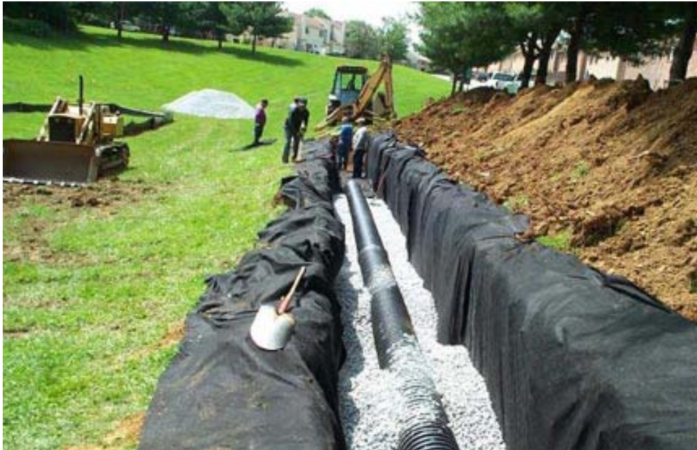
Figure A8. Construction of infiltration trench. (Used with permission.)
