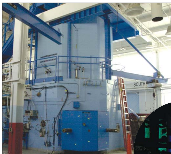
A biological shield, center, surrounds the core of the tank-type reactor in which primary coolant was used for cooling the reactor's core. Inset photo: Cherenkov radiation, when it is intense, appears as a weak bluish-white glow in the pools of water shielding the nuclear reactor. The Cherenkov radiation is caused by electrons from the reactor traveling at speeds greater than the speed of light in water, which is 75 percent of the speed of light in a vacuum. Top photo by LeRoy N. Sanchez; inset photo by Jose "Mitzie" Ulibarri, former Information Services (IS-7)
