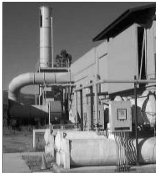
The new Beryllium Technology Facility, has a state-of-the-art exhaust system. Below: The ventilation system changes the air up to 15 times an hour.
