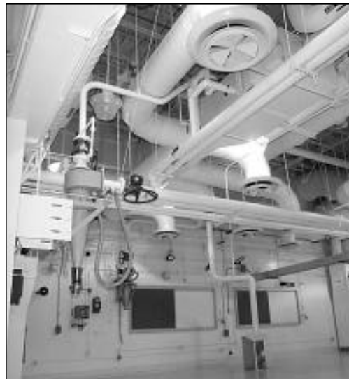
The new Beryllium Technology Facility, has a state-of-the-art exhaust system. Below: The ventilation system changes the air up to 15 times an hour.
