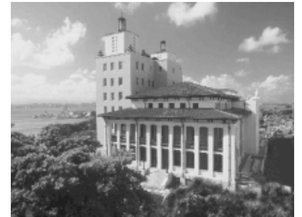
A 2002 award winner in the General Services Administration's Design Awards was the rehabilitation of the 1914 U.S. Post Office and Courthouse in Old San Juan, Puerto Rico. These awards honor the best projects designed and constructed by the agency, with professional private-sector peers selecting the entries. (Photo courtesy of the General Services Administration)
