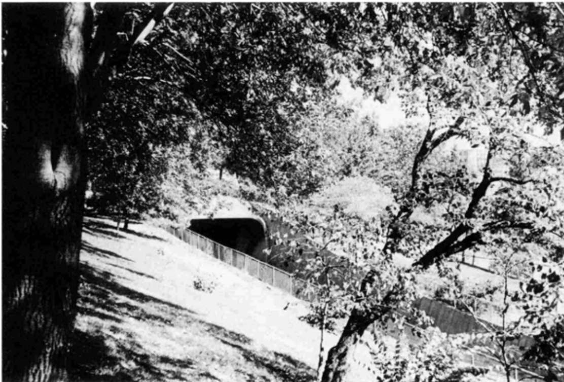
Figure 75: Chain-link fence surrounding railroad cuts, (Chan, 1996).
